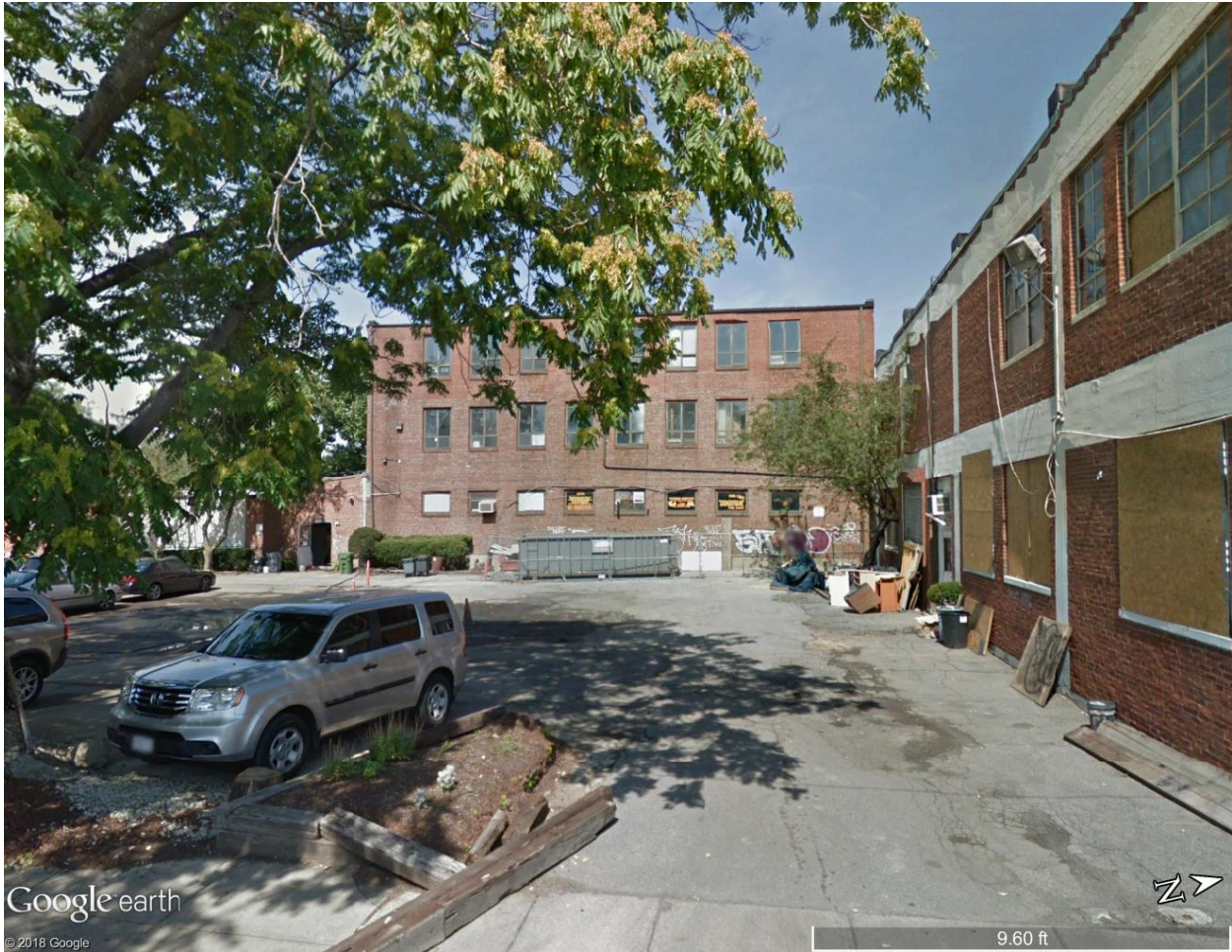
STREET VIEW OF SITE LOOKING WEST ON EMERY ROAD
