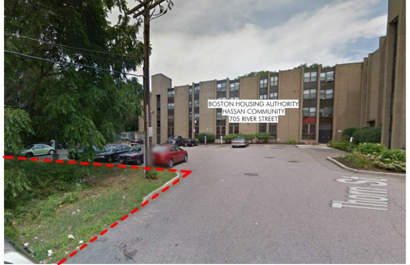
VIEW 3 HOUSING AUTHORITY BUILDING ADJACENT TO SITE
