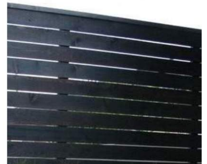
SITE FENCE Horizontal board fence along MBTA Embankment and at Trash Enclosure
