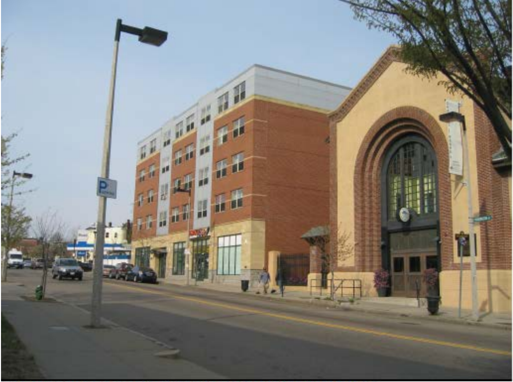
WASHINGTON ST. 5 STORY MIXED USE BLDG AND BNN CABLE BLDG
