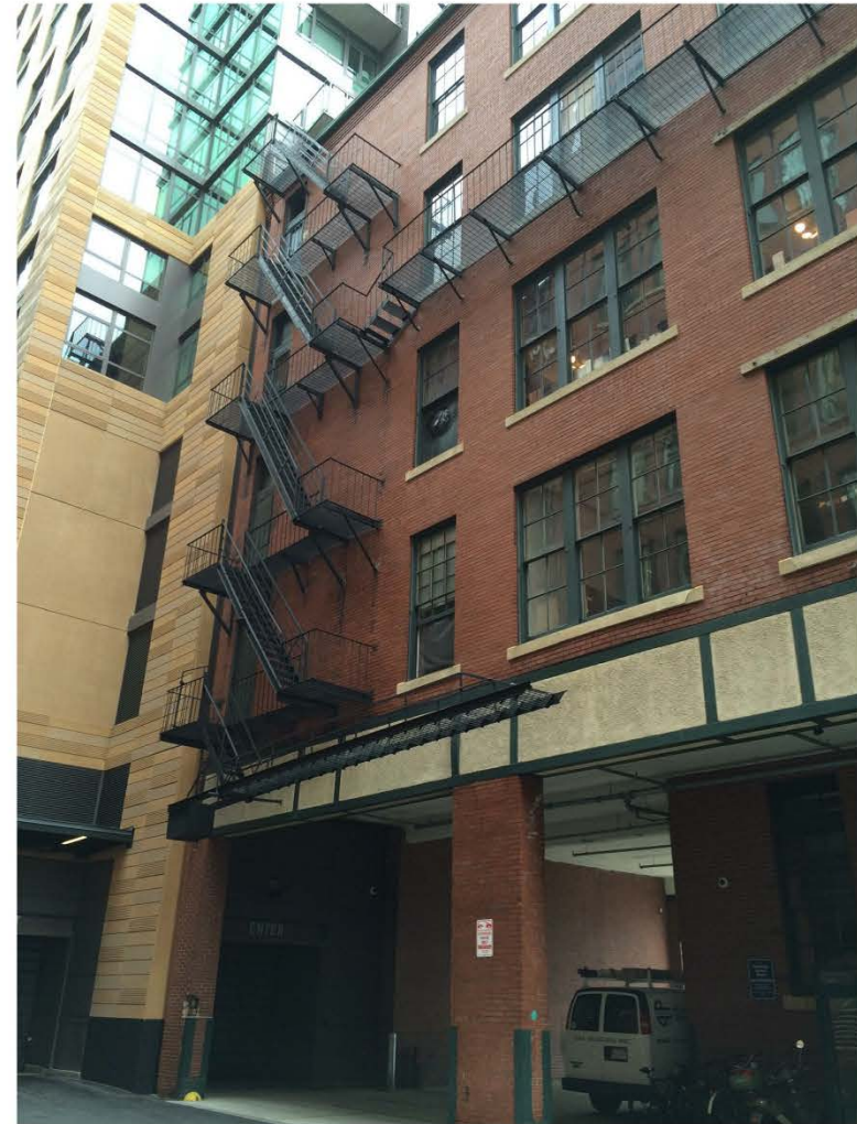
EXISTING FIRE ESCAPE LADDER
