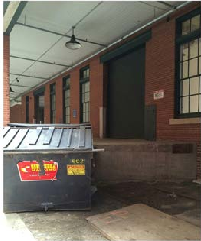
EXISTING LOADING AREA
