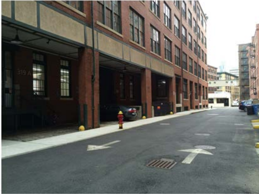
EXISTING LOADING AREA
