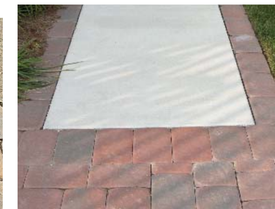
Concrete sidewalk with permeable paver border
