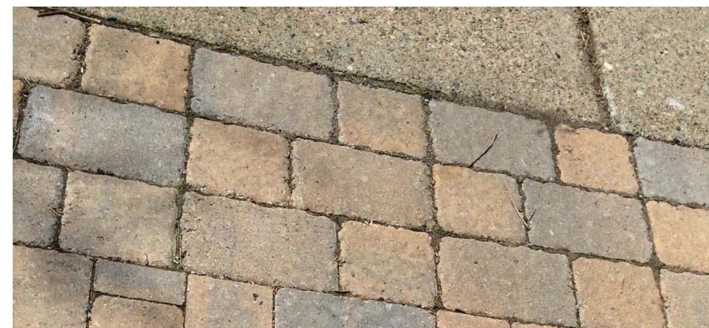
Permeable pavers flush with asphalt
