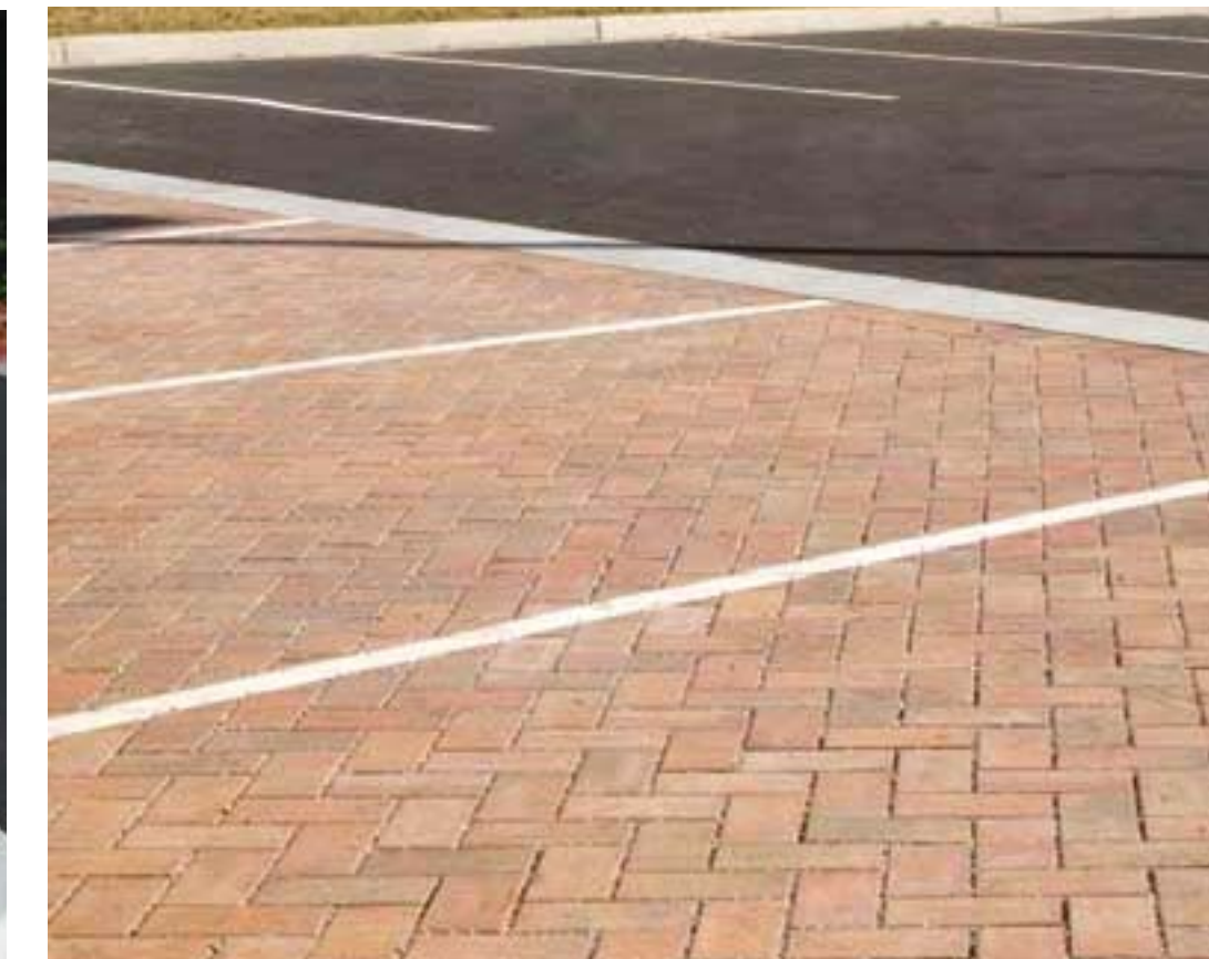
Permeable pavers flush with asphalt
