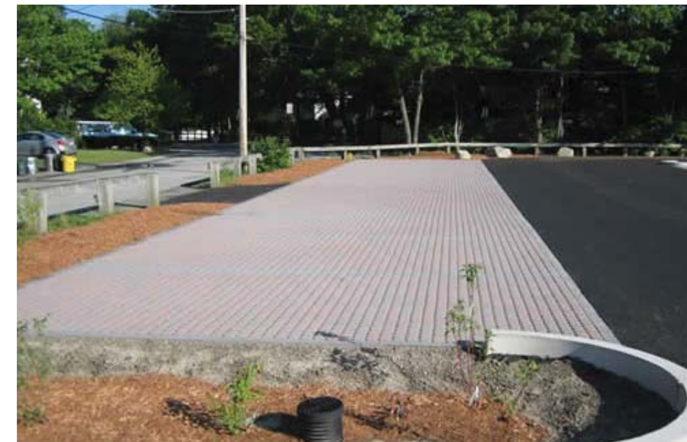
Permeable pavers flush with asphalt
