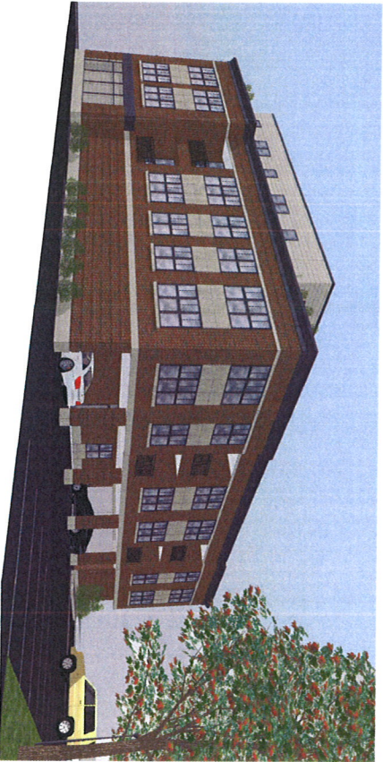
VIEW FROM NORTHEAST CORNER ALONG REAR PROPERTY LINE
