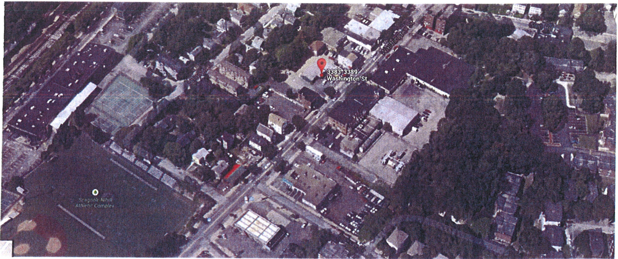
Bird's eye view of 3385-3389 Washington Site from the south
