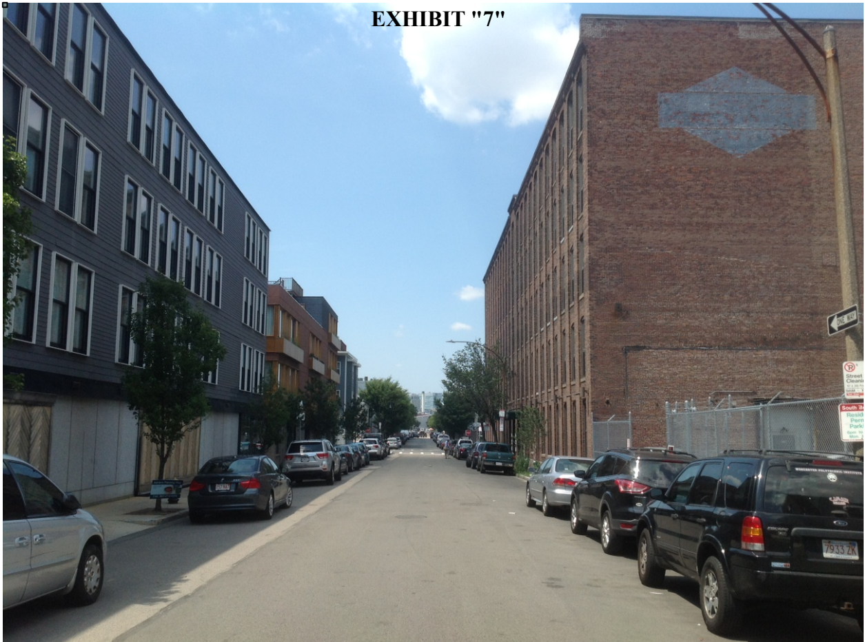
VIEW DOWN WEST SECOND STREET TOWARDS "E" STREET
