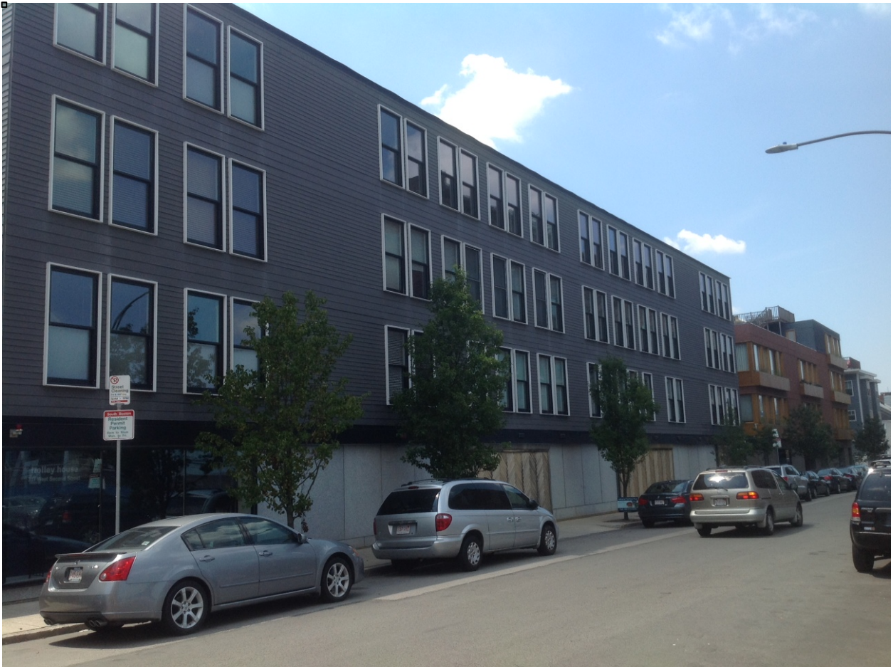
VIEW OF TROLLEY HOUSE BUILDING ACROSS WEST SECOND STREET
