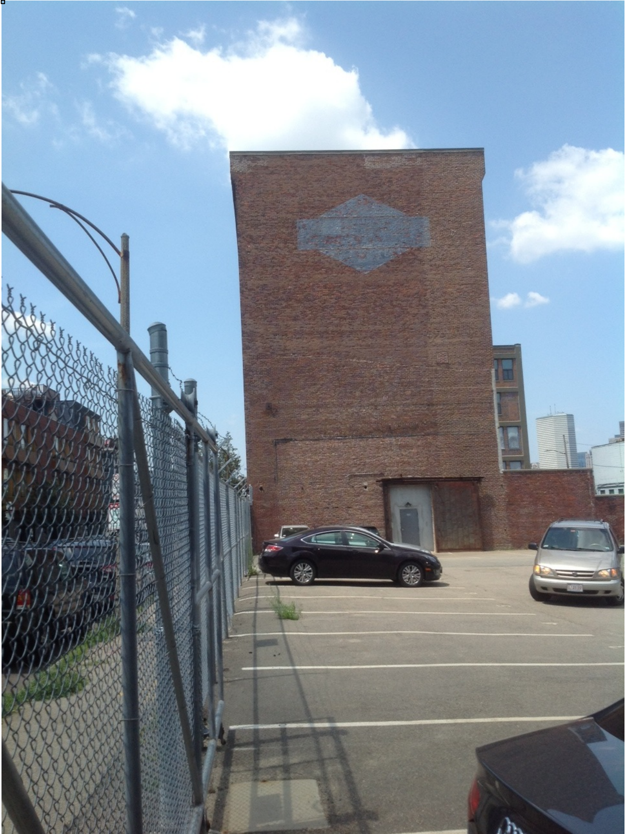
VIEW OF LOCUS ALONG WEST SECOND STREET, FOUNDRY BUILDING IN BACKGROUND
