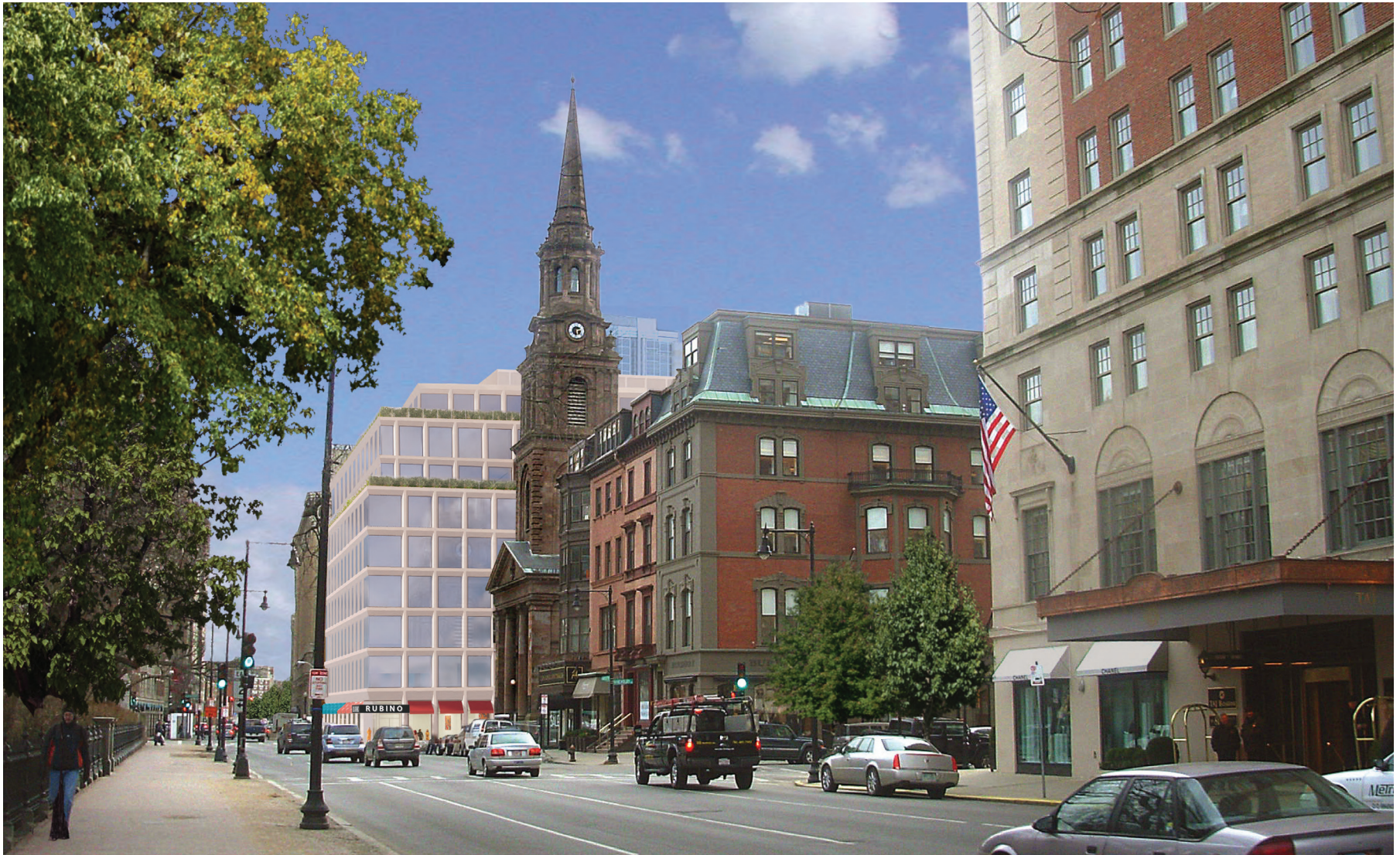
VIEW LOOKING SOUTH ON ARLINGTON STREET
