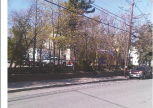
EXISTING WALLS ALONG ASHFORD STREET
