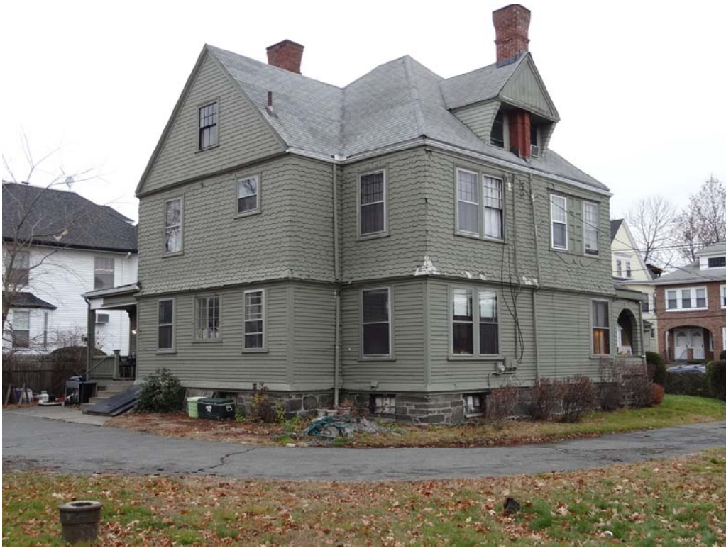
SOUTH WEST VIEW OF EXISTING HOUSE
