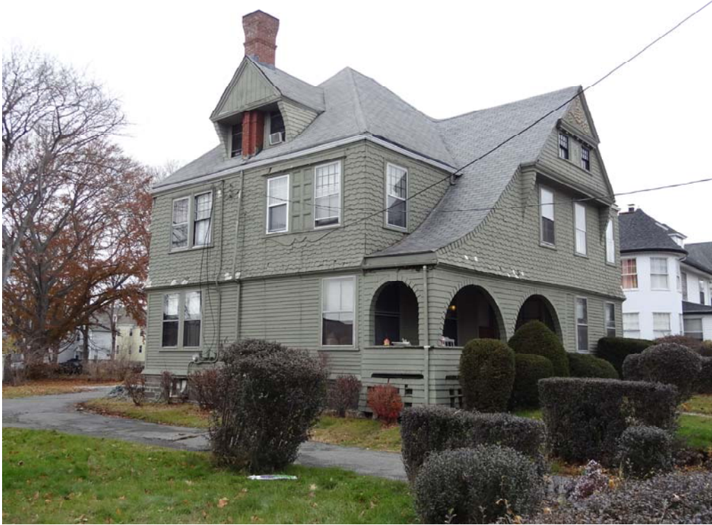
SOUTH EAST VIEW OF EXISTING HOUSE (FROM PARSONS STREET)
