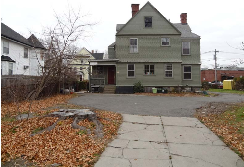
BACK OF EXISTING HOUSE
