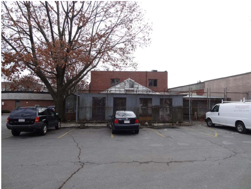
EXISTING PARKING LOT
