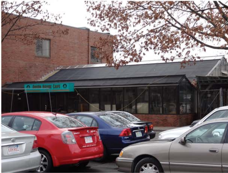
EXISTING BUILDING (ON SITE)
