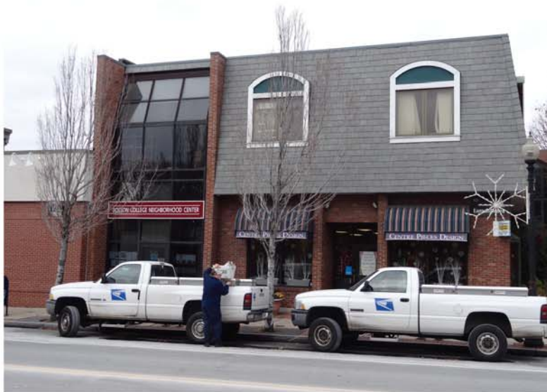
EXISTING BUILDING (ON SITE)
