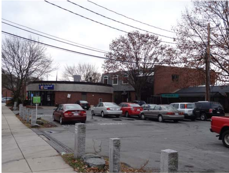
EXISTING BUILDING (ON SITE)
