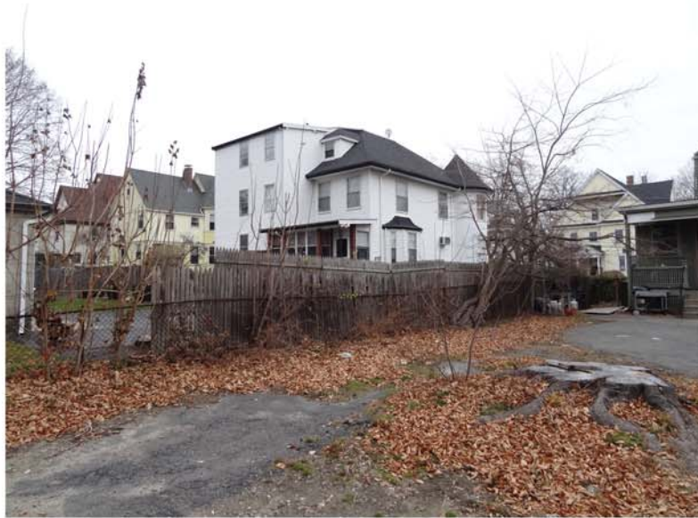
EXISTING BUILDING (RIGHT)
