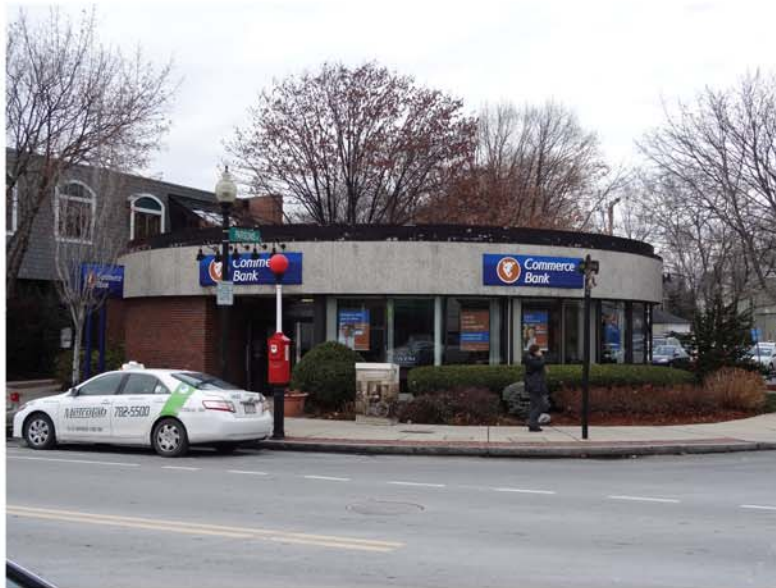
EXISTING BUILDING (ON SITE)
