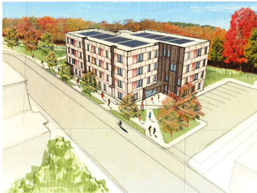
AERIAL VIEW FROM NEW ENGLAND AVE
