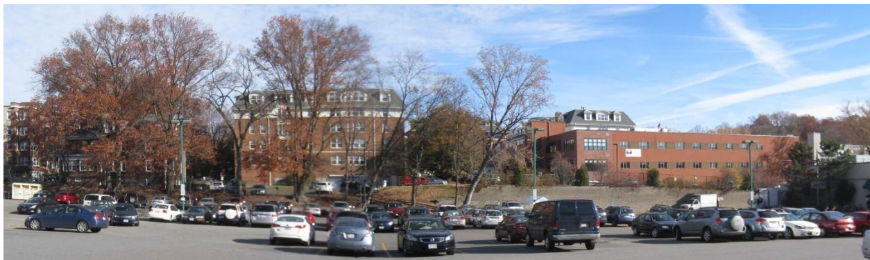
Boston 5 Story Nursing Home – “Brighton House”
