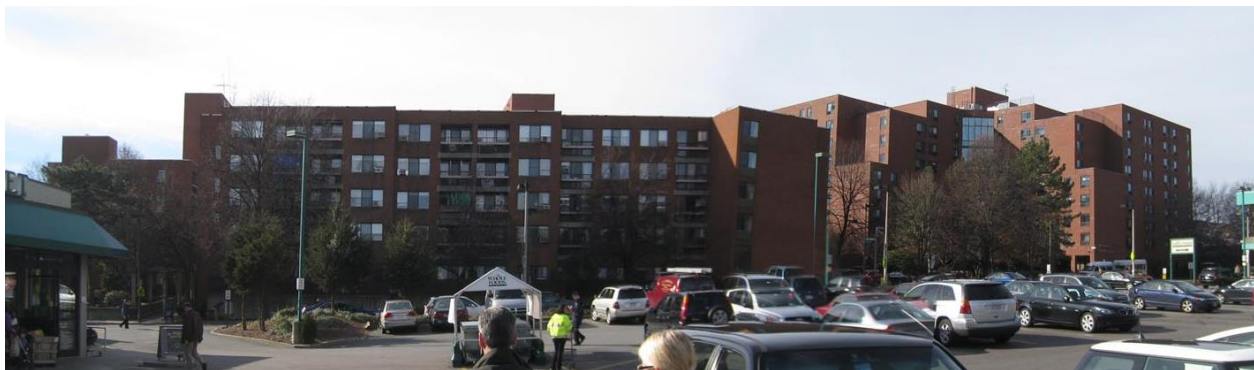
Boston 5-9 Story Brick Buildings – “Patricia White Apartments” and “B’nai B’rith Housing”
