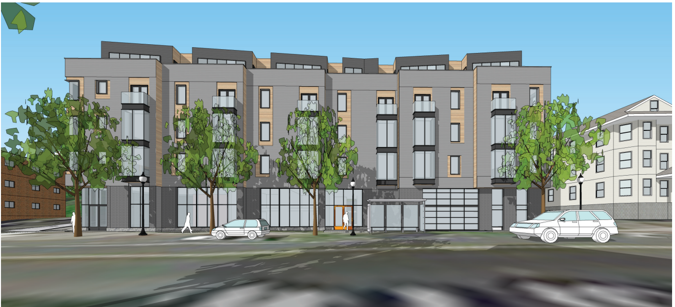
Figure 3: North view along Washington St.
