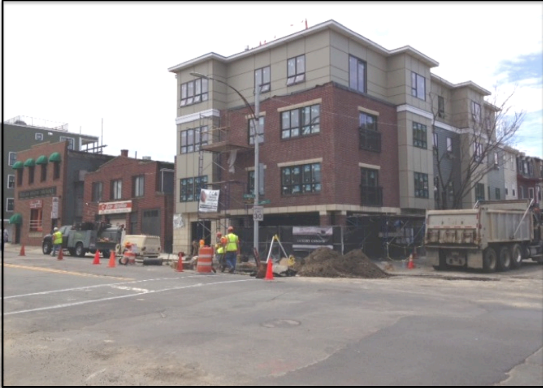
NEW CONSTRUCTION AT CORNER OF L AND EAST SECOND STREET
