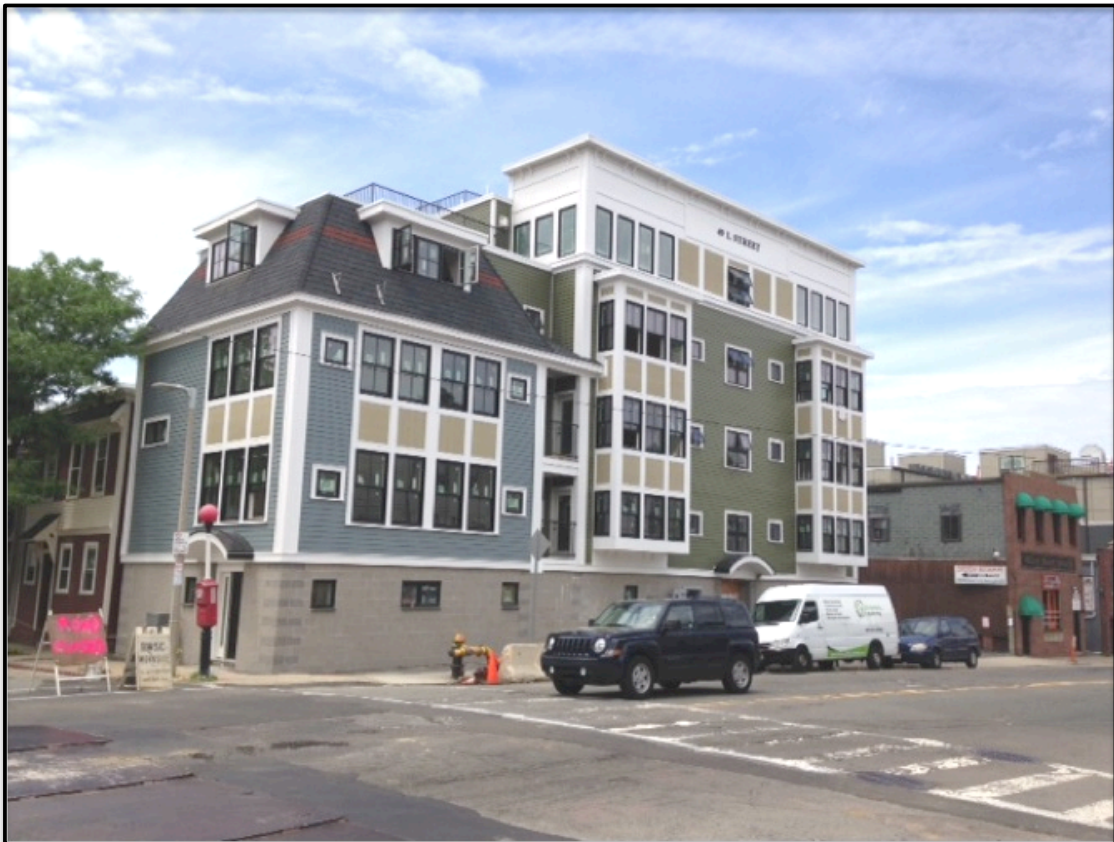
NEW CONSTRUCTION AT CORNER OF L AND EAST THIRD STREET
