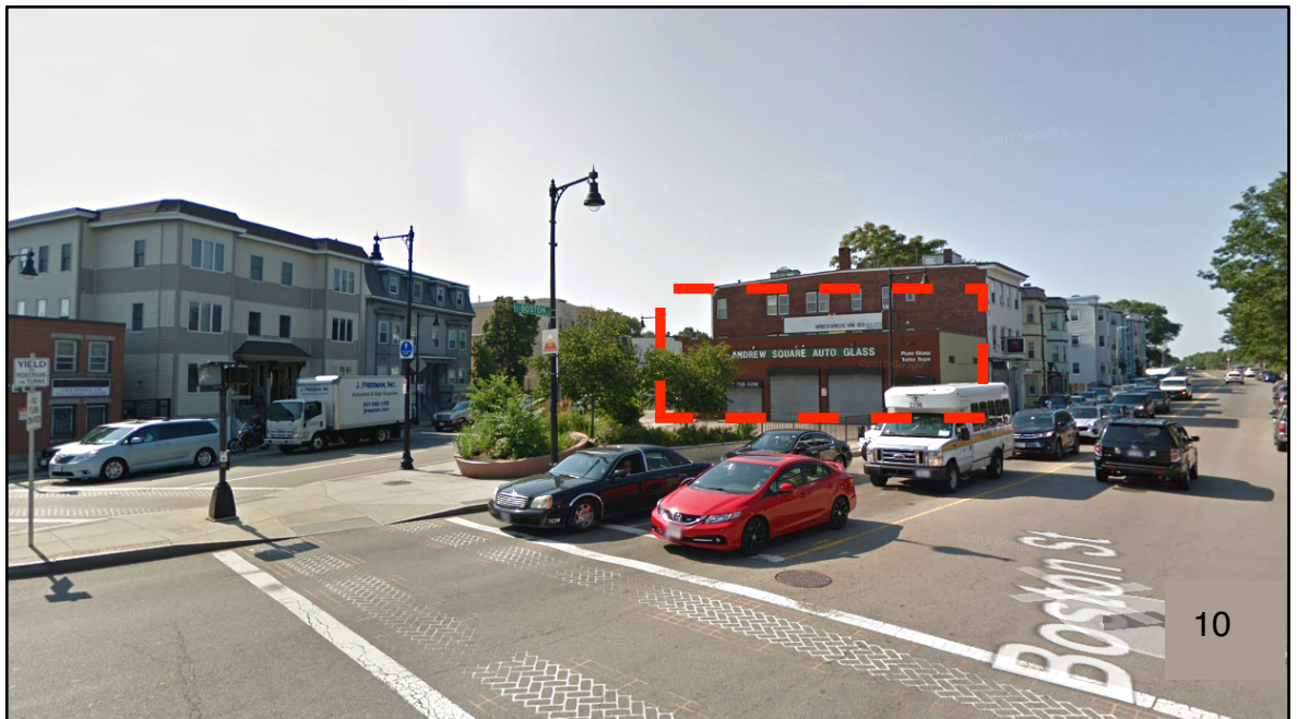
View of Site from Boston Street
