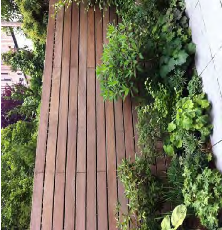
Fence (42" ht. for fall guard) on Wall
