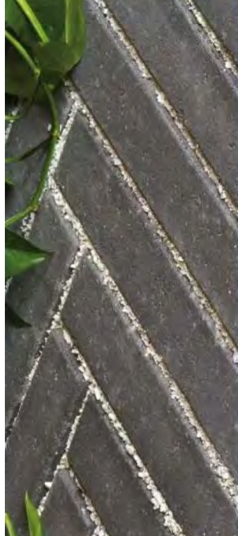
Permeable Pavers define the Rear Yard Terrace allowing infiltration of storm water
