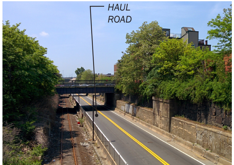
VIEW DOWN HAUL ROAD TOWARDS SITE
