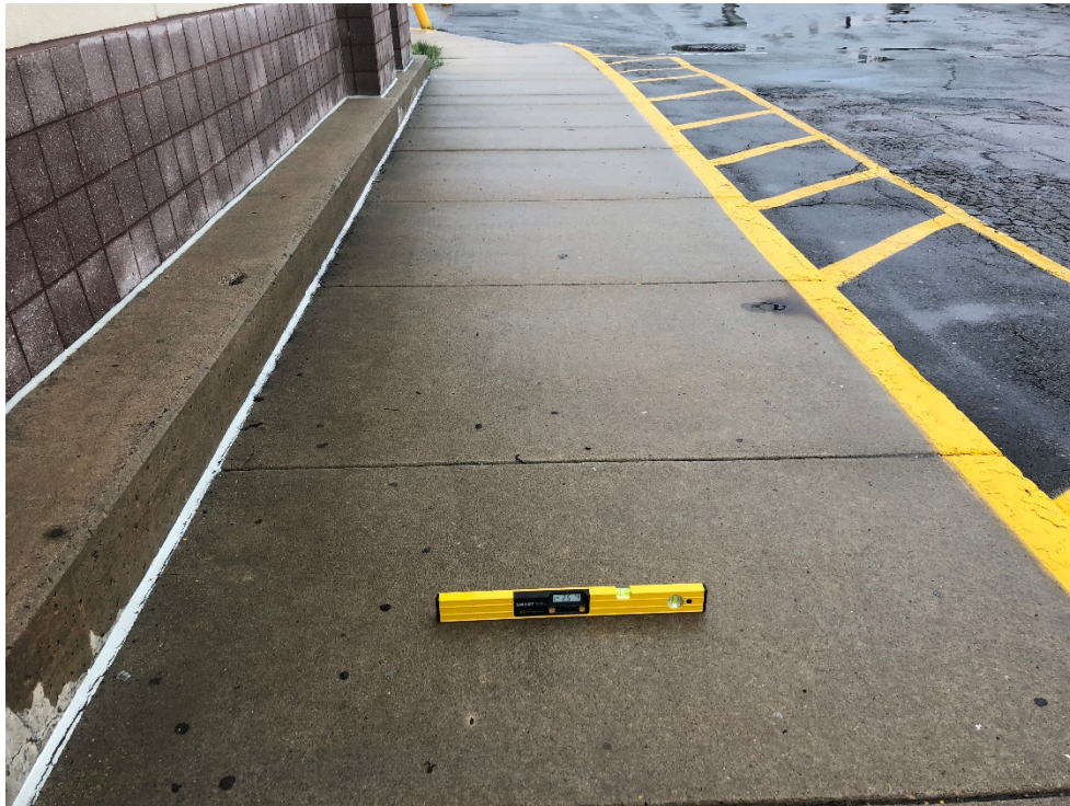
Figure 3.3: Existing Sidewalk with 2.5% Cross-Slope (2.0% Max. Allowed)
