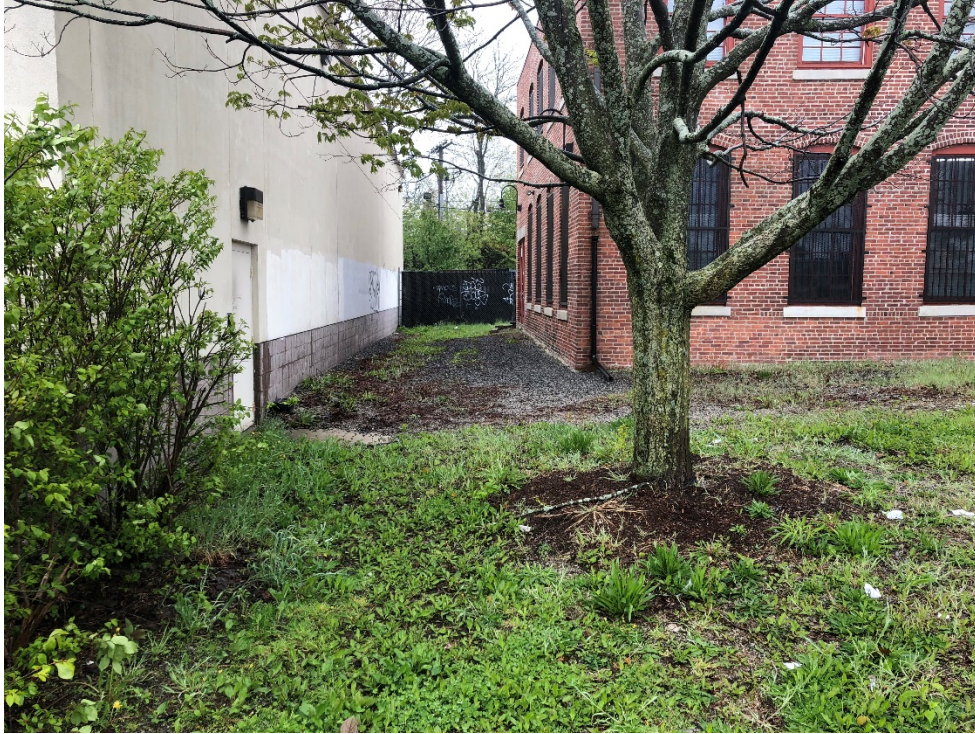
Figure 3.5: Existing Compactor Location (Rear)
