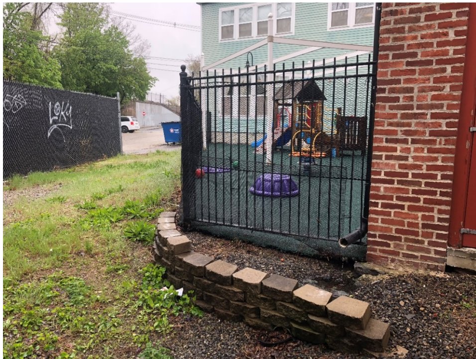
Figure 3.6: Existing Compactor Location (Left)
