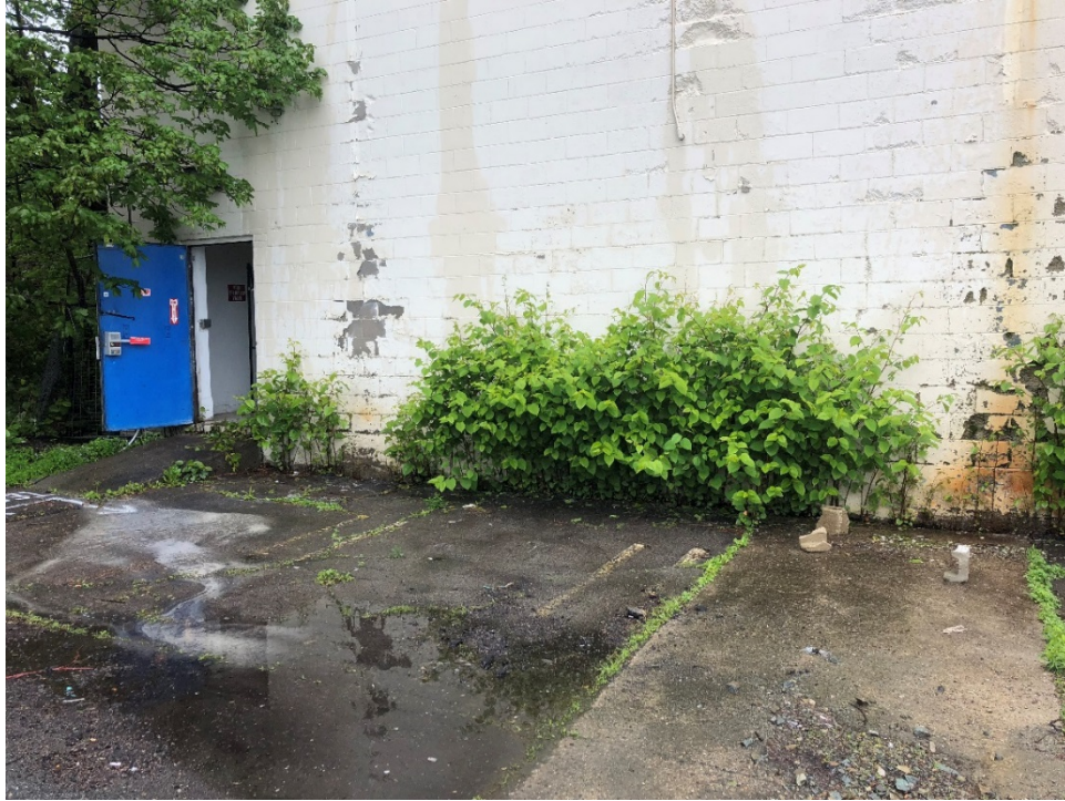
Figure 3.9: Existing Southeast Building Façade
