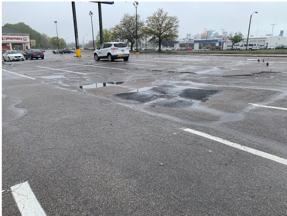
Figure 3.10: Existing Catch Basin in Parking Area
