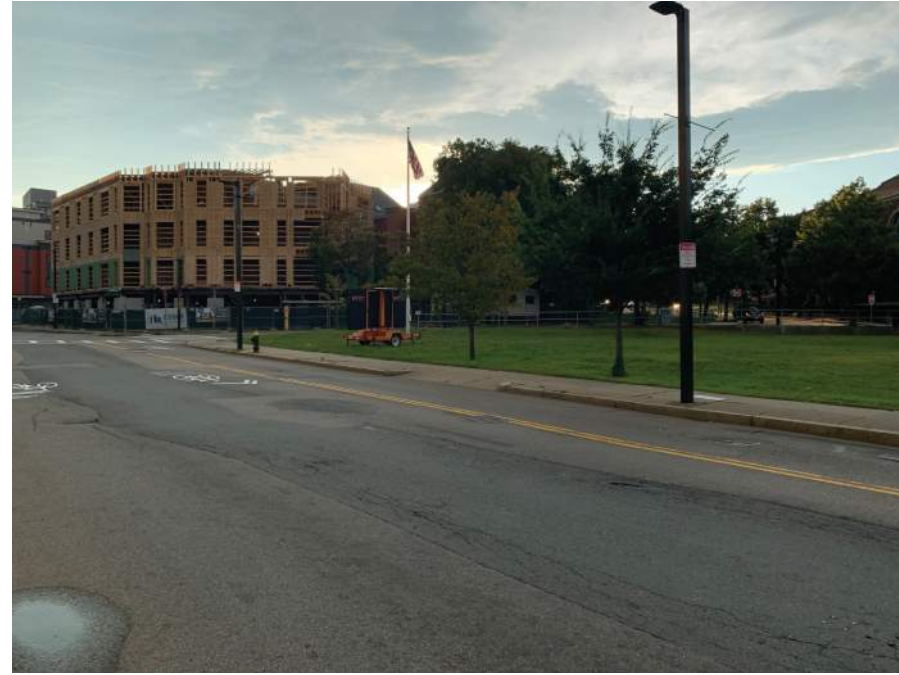
2 ADJACENT BUILDING - 2451 WASHINGTON ST.
