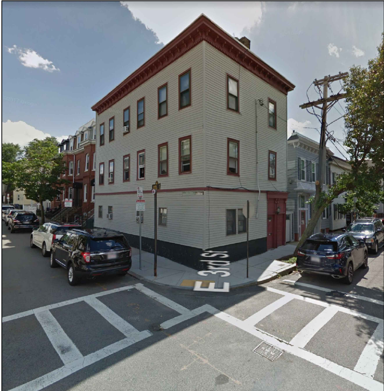
INTERSECTION OF EAST THIRD STREET AND P STREET
