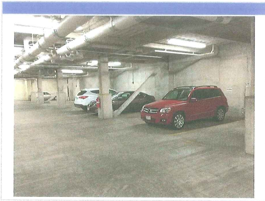
Garage in Adjacent Building
