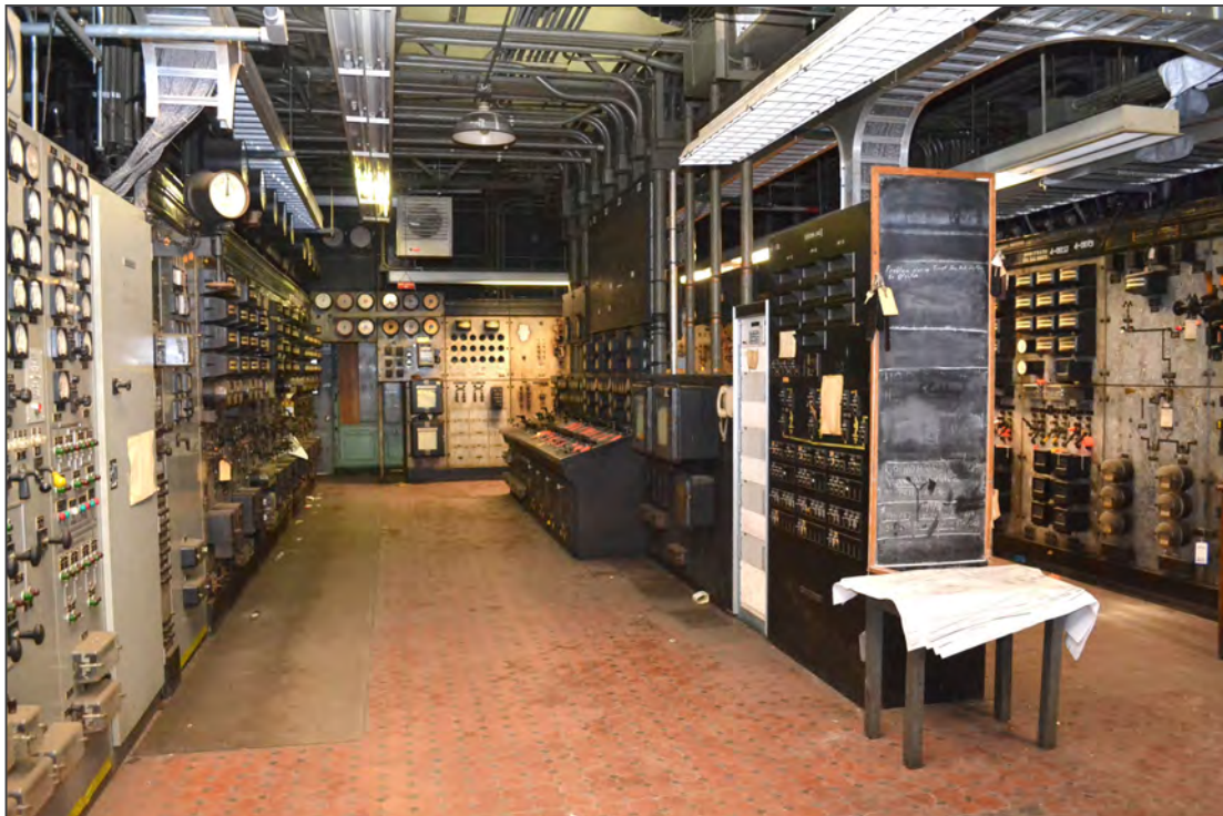
28. Switch House, facing south
