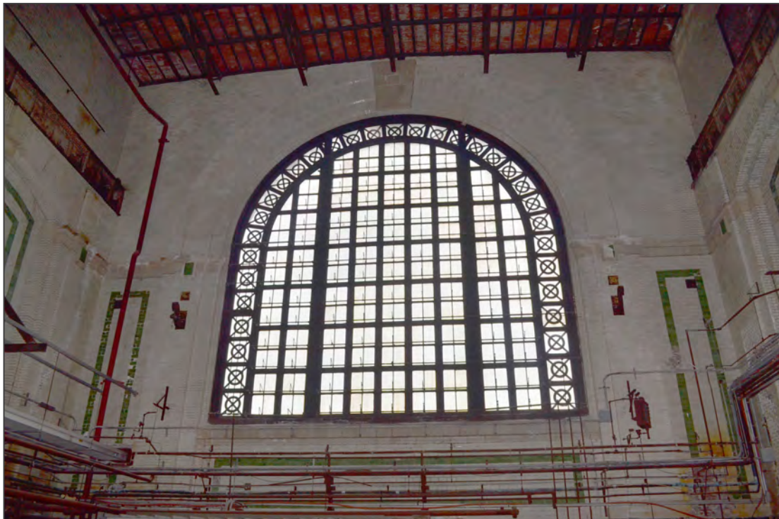
16. 1898 Turbine Hall, facing north
