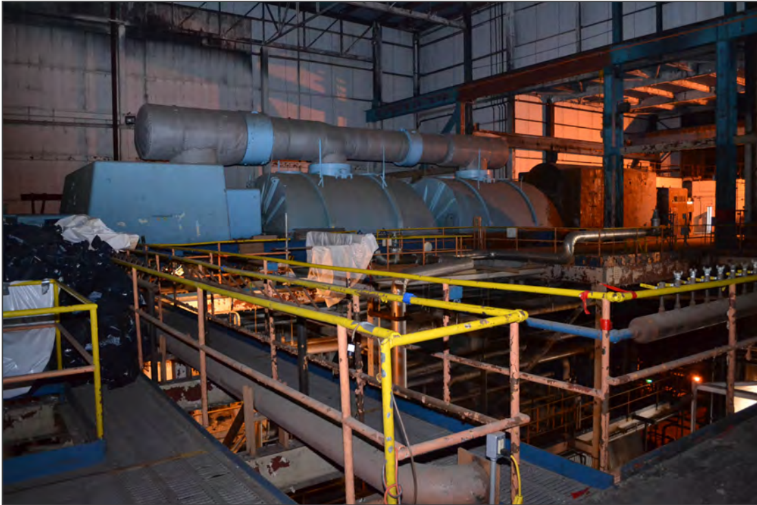
5. Turbine Hall No. 1, facing southeast
