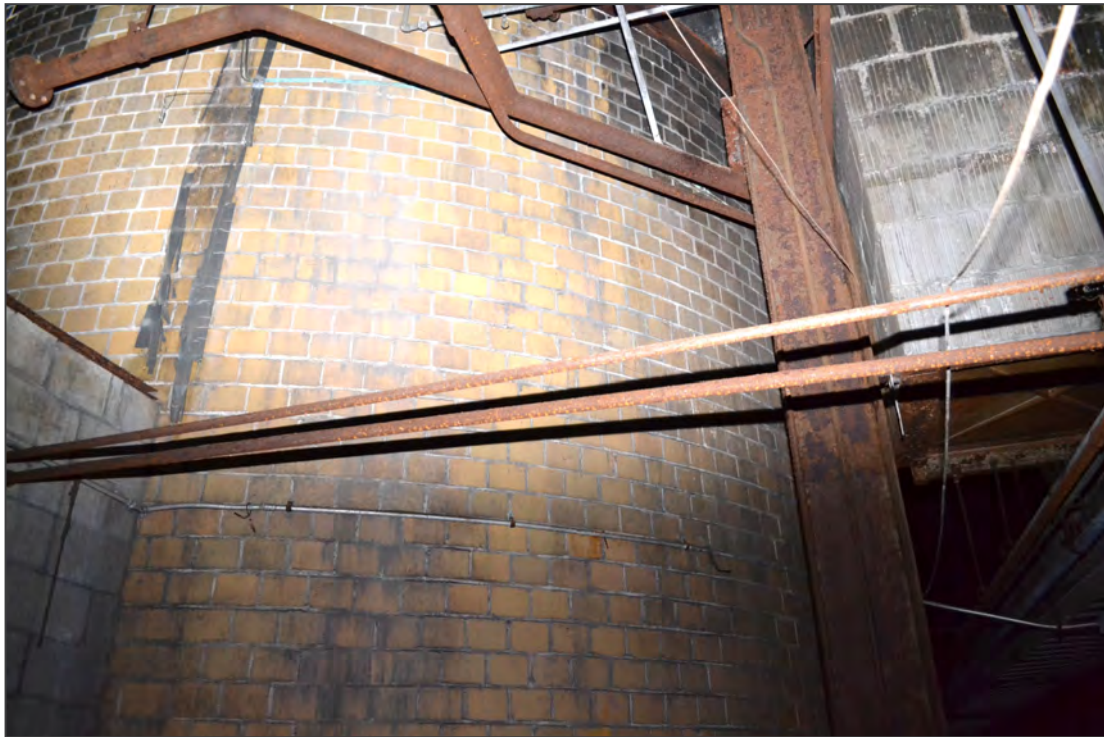
9. Turbine Hall No. 3, facing southeast
