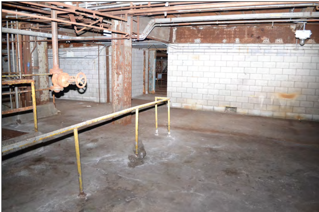
10. Turbine Hall No. 3, facing southwest
