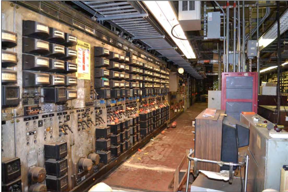
23. Switch House, facing south
