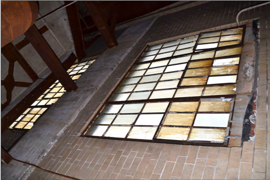
13. Turbine Hall No. 3, facing southwest
