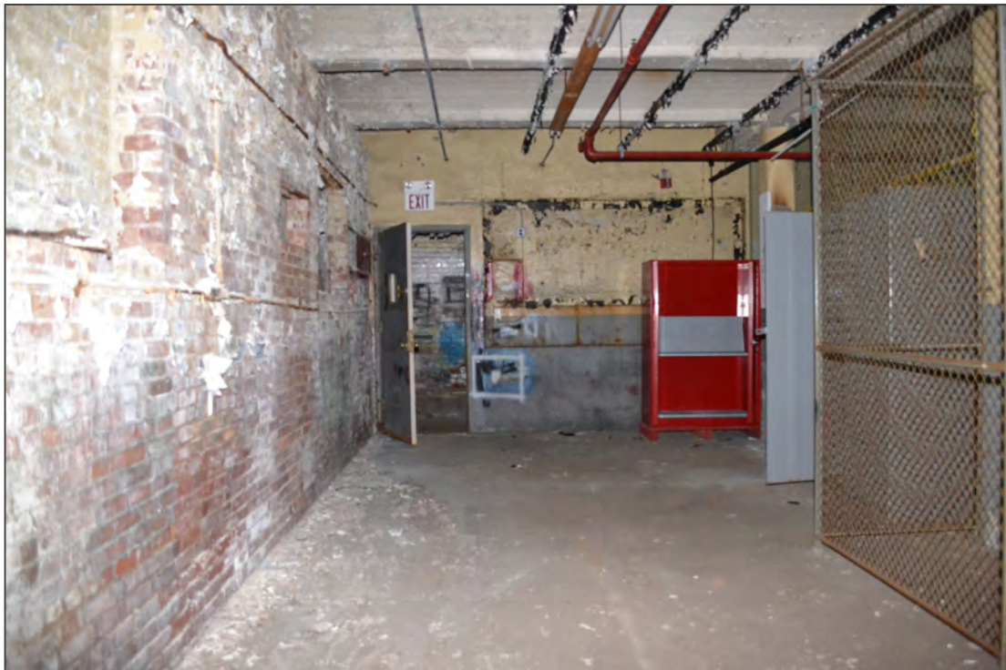
22. Boiler Room, facing south
