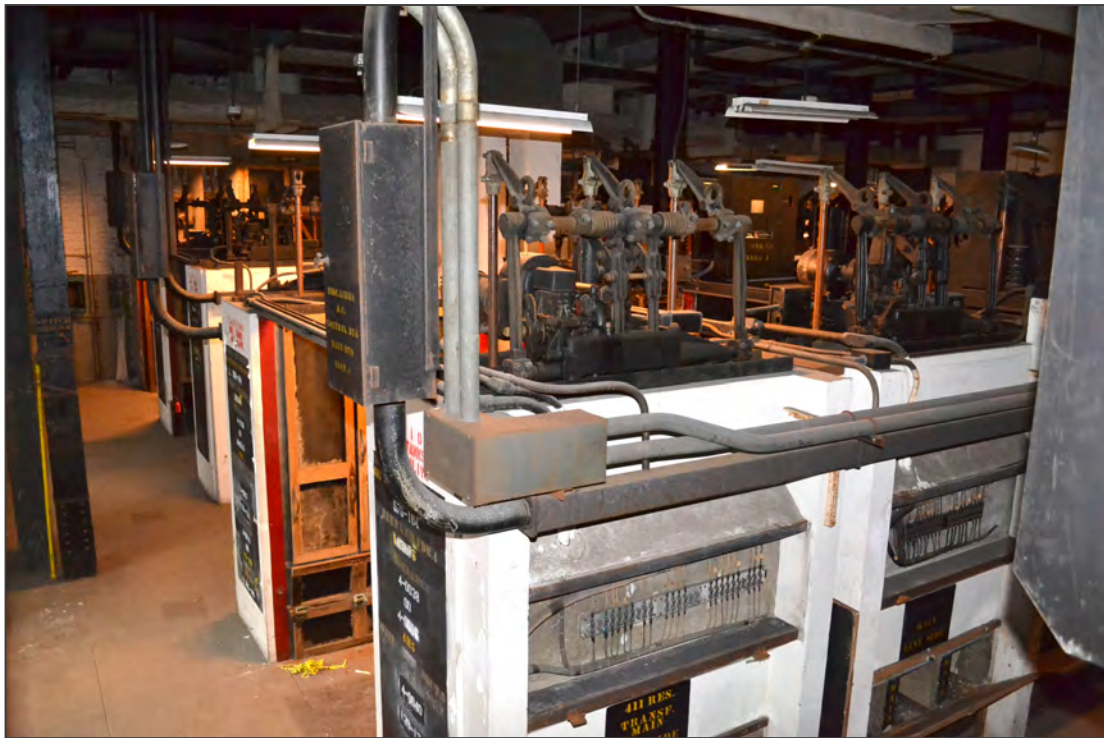
24. Switch House, facing northeast
