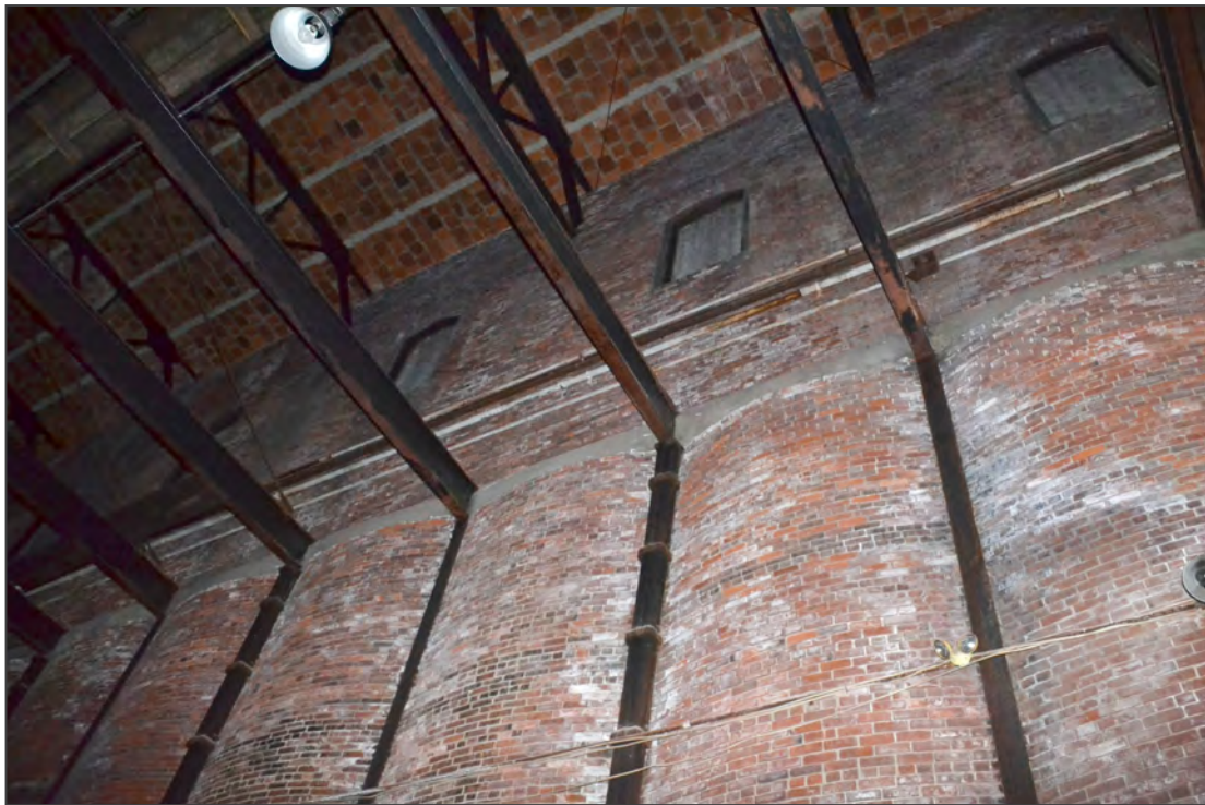
30. Coal Pit detail
