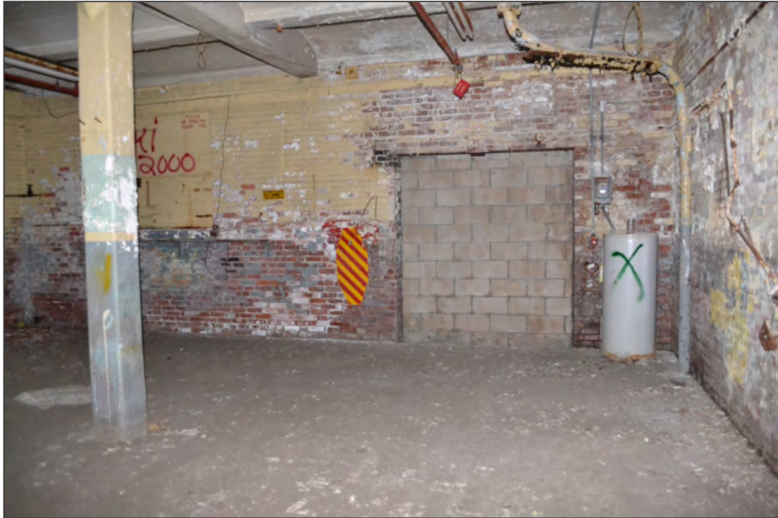
21. Boiler Room, facing north
