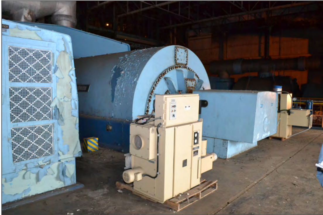
3. Turbine Hall No. 1, facing southwest
