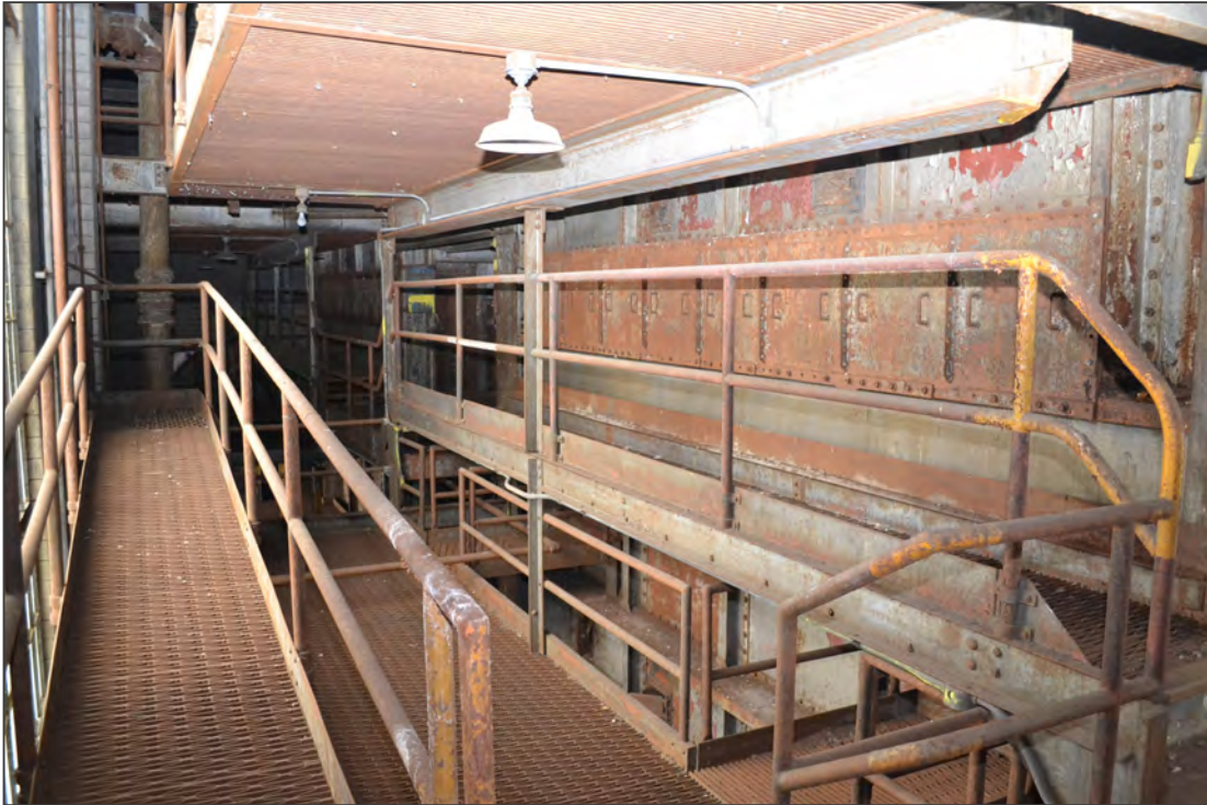
7. Turbine Hall No. 1 basement, facing northeast
