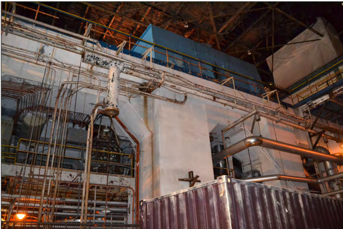
2. Turbine Hall No. 1, facing southeast
