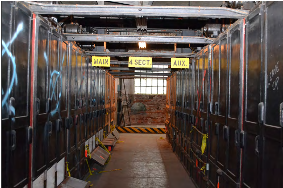
25. Switch House, facing south
