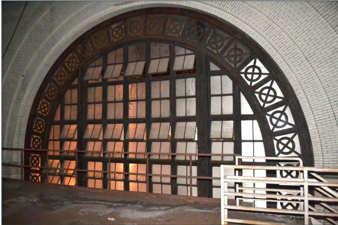
19. 1898 Turbine Hall, facing north
