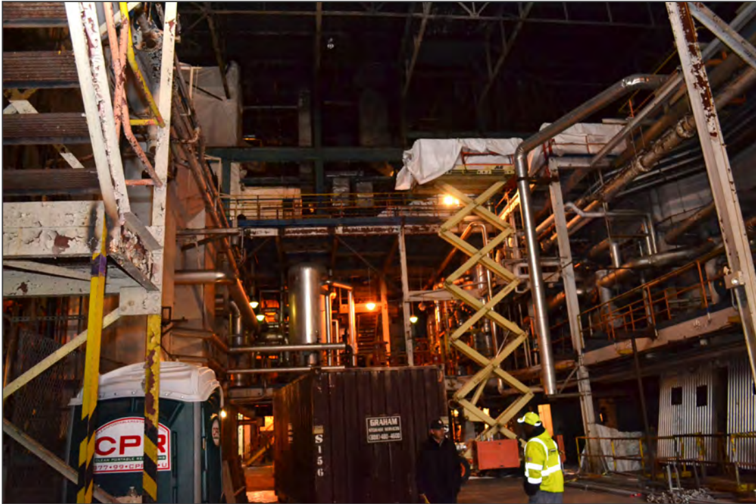
1. Turbine Hall No. 1, facing south
