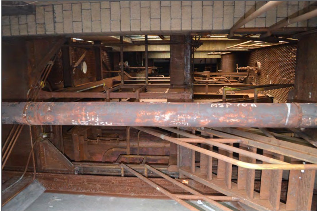
11. Turbine Hall No. 3 basement, facing east
