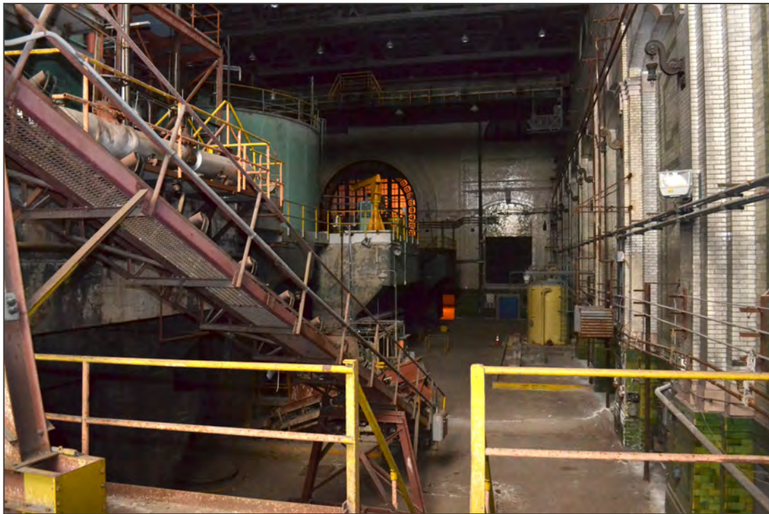
18. 1898 Turbine Hall, facing north
