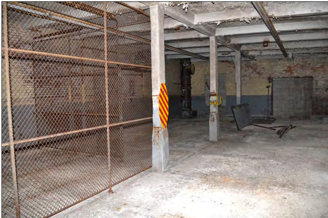
20. Boiler Room, facing northwest
