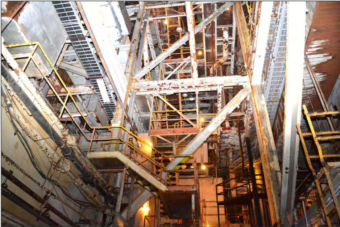
8. Turbine Hall No. 2, facing south
