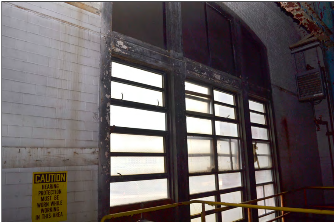
4. Turbine Hall No. 1, facing northeast
