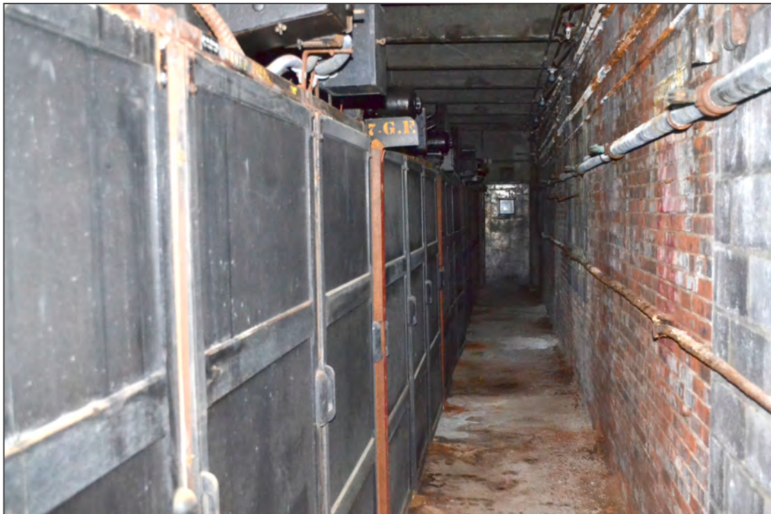
26. Switch House basement, facing north
