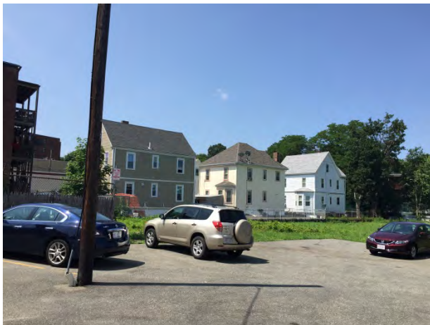
SITE WITH REAR OF TILMAN STREET BUILDINGS
