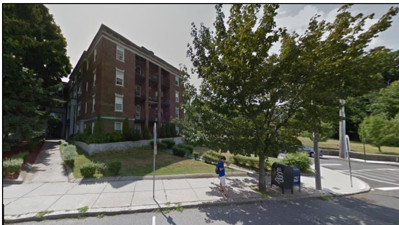
2. View of 45 Chestnut Hill Ave (north).
