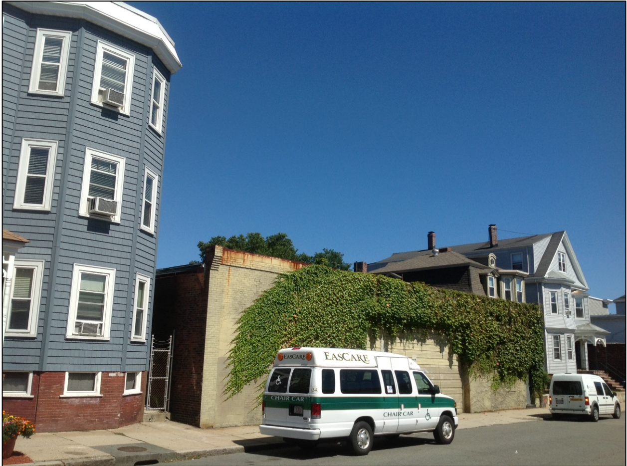
EXHIBIT 7 - ALTERNATE VIEW OF SITE, EAST SIXTH STREET SIDE
