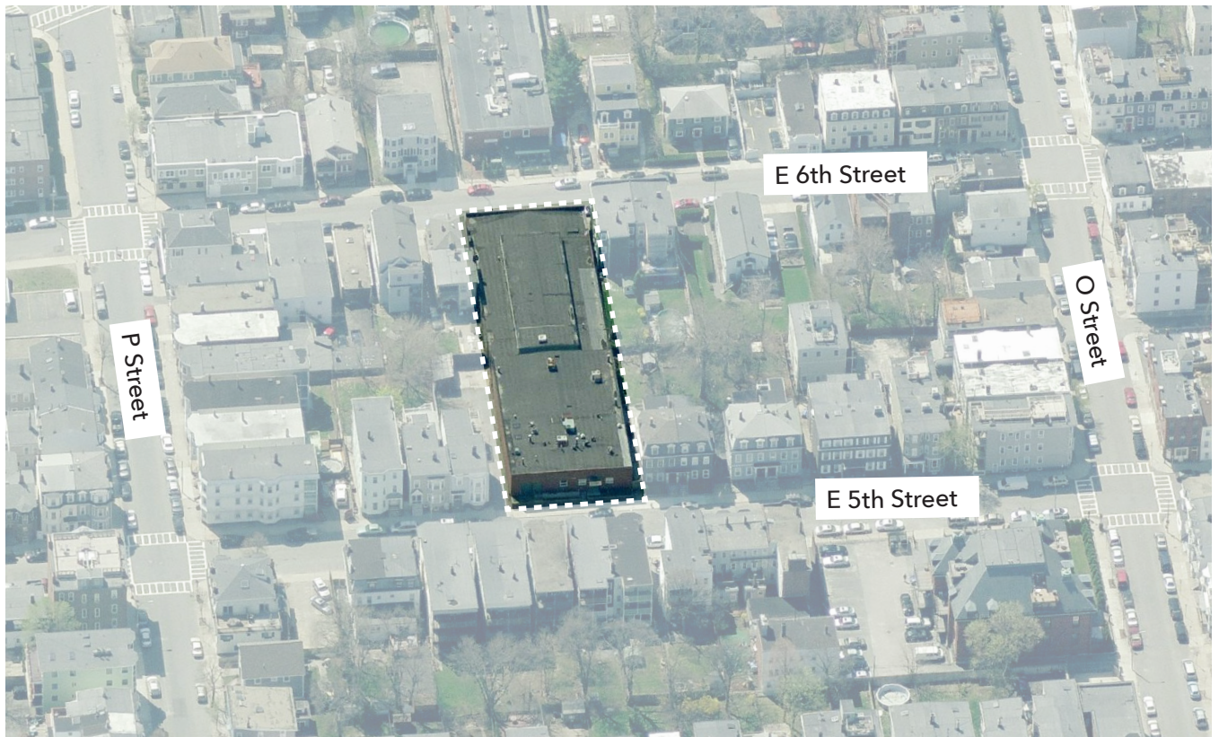
EXHIBIT A AERIAL VIEW FROM NORTH
