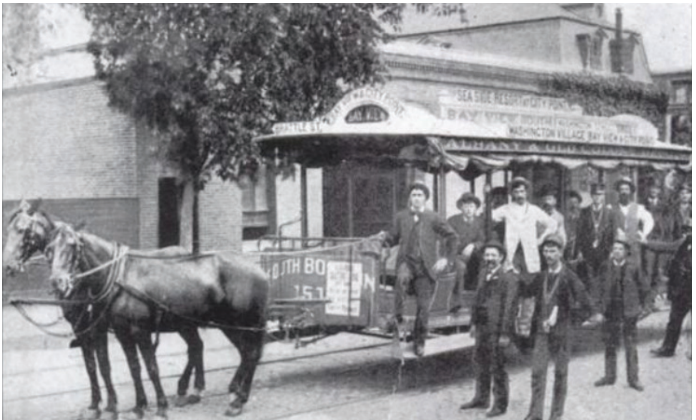
PHOTOGRAPH OF EXISTING BUILDING, 1884
