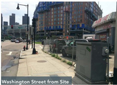
Washington Street from Site
