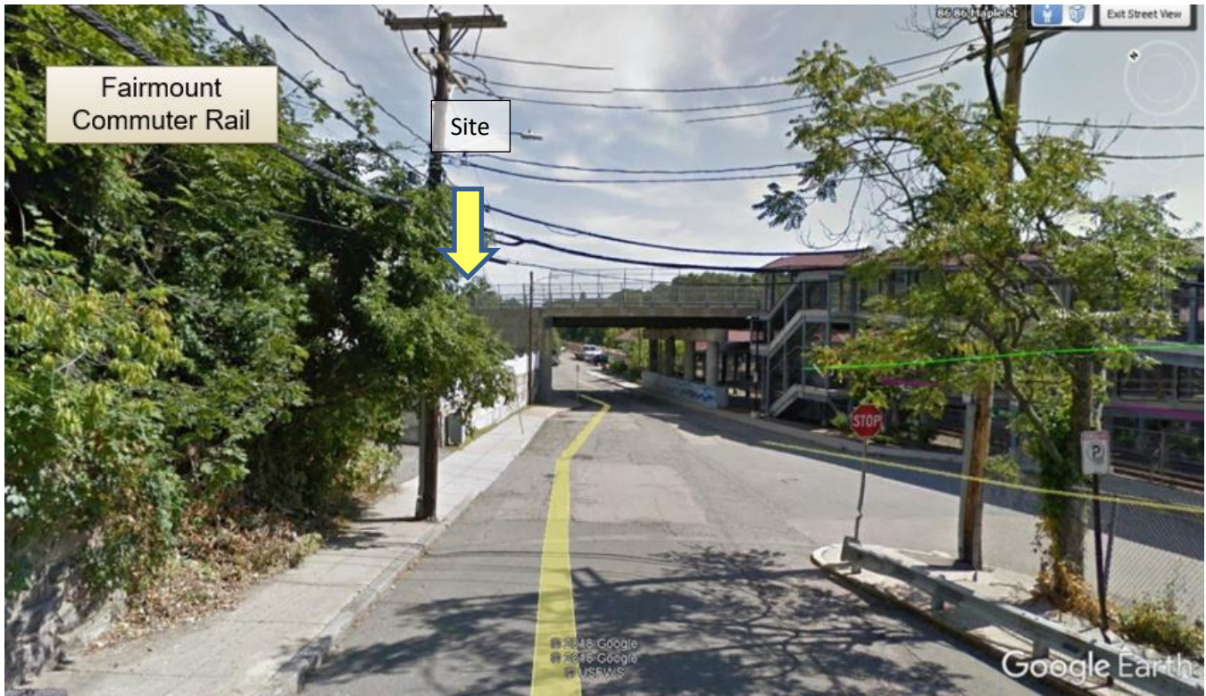
Fairmount Commuter Rail Station looking north from Maple Street
