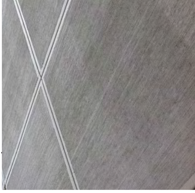
Concrete Sidewalk, Simple and well maintained.
