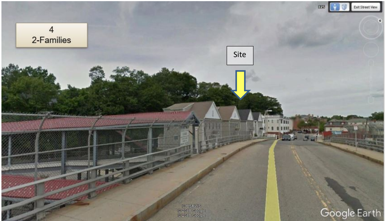
Proposed project site looking northwest on Fairmount Avenue.
