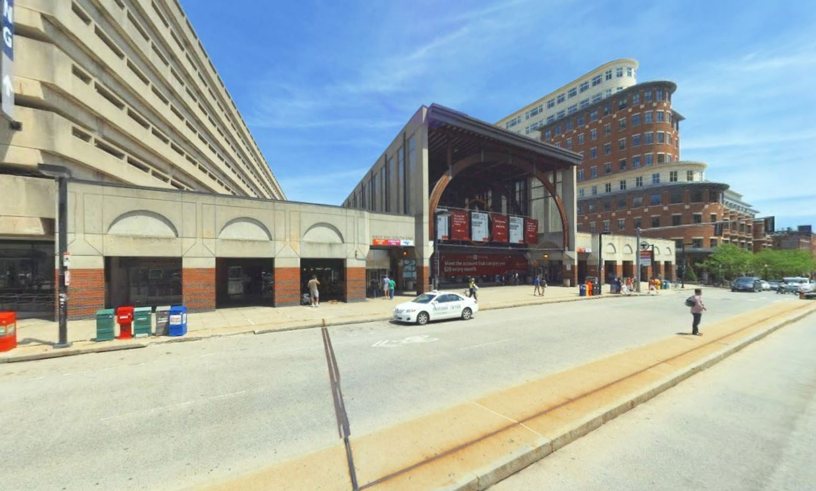
VIEW FROM DARTMOUTH STREET - EXISTING CONDITION
