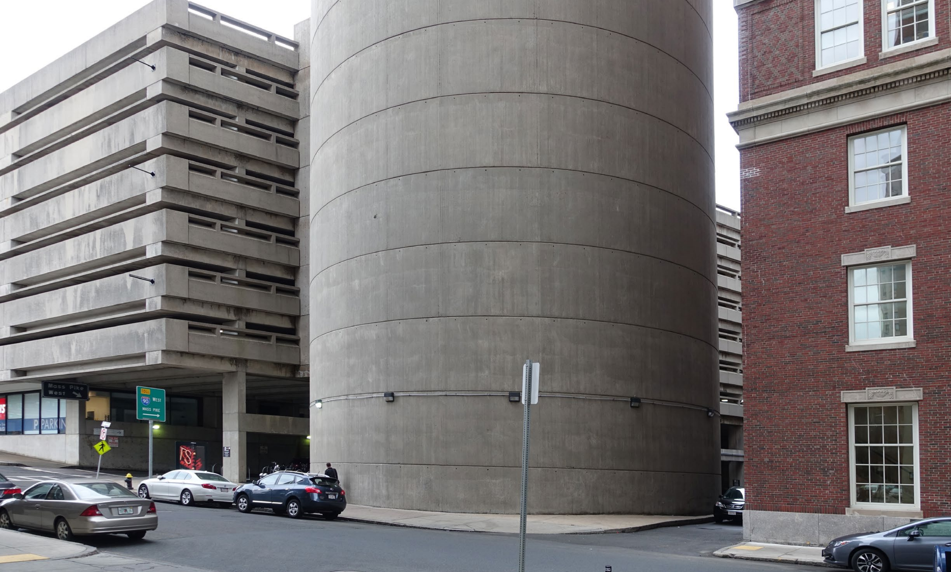
VIEW OF GARAGE EAST STREET LEVEL - EXISTING CONDITION
