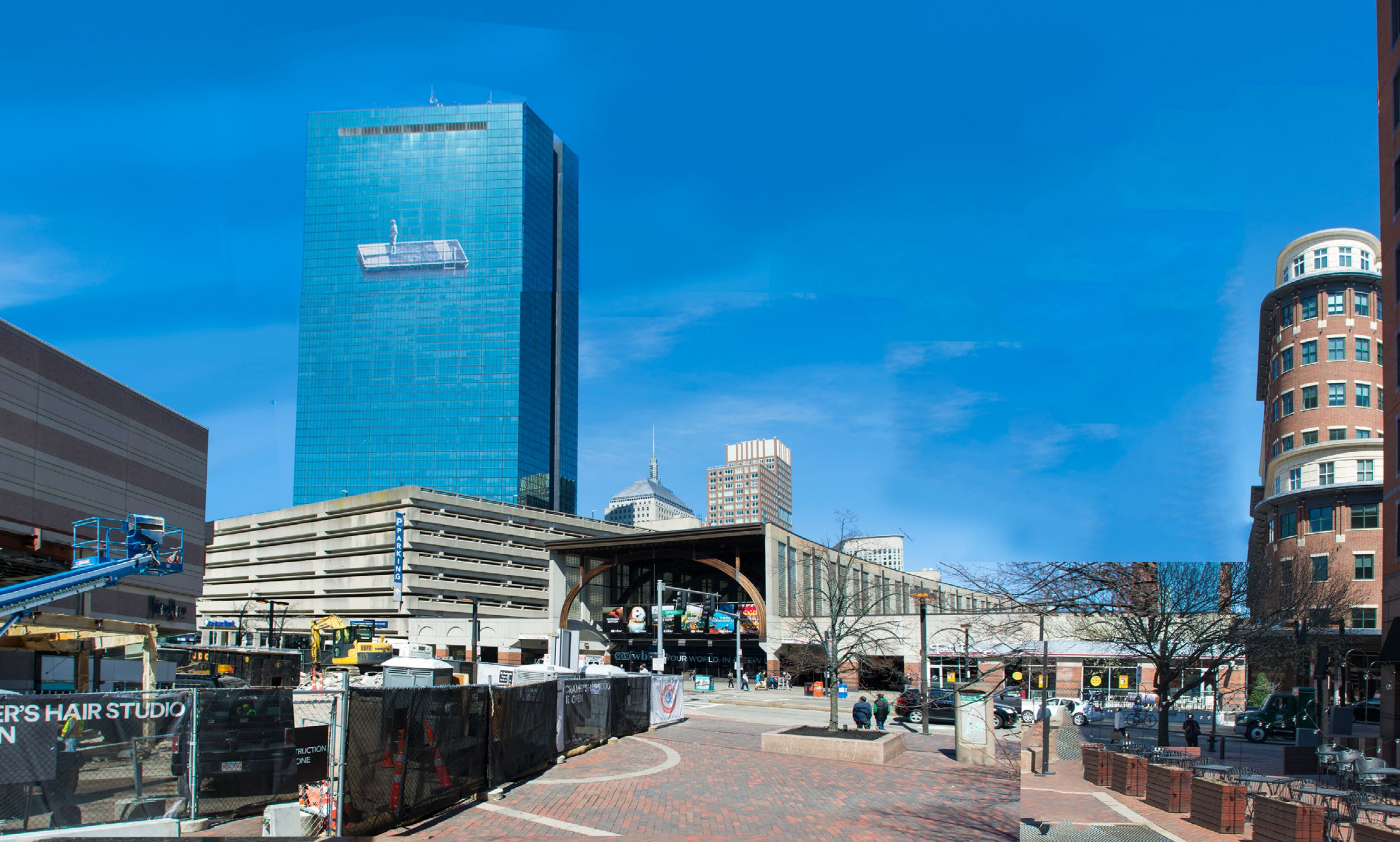
VIEW FROM SOUTHWEST CORRIDOR - EXISTING CONDITIONS
