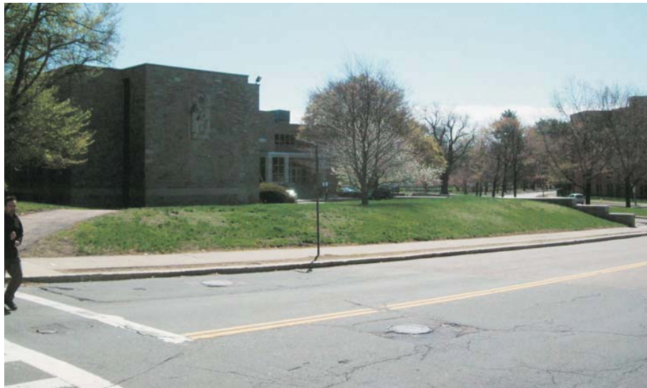
View looking Southeast from Commonwealth Avenue/ St. Thomas More Road Intersection
