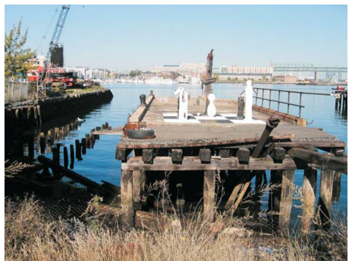
View of piers looking west
