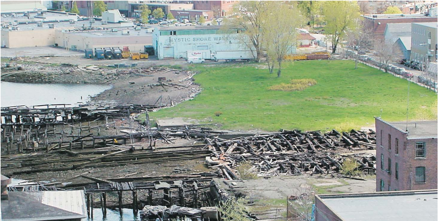
View of project site looking north
