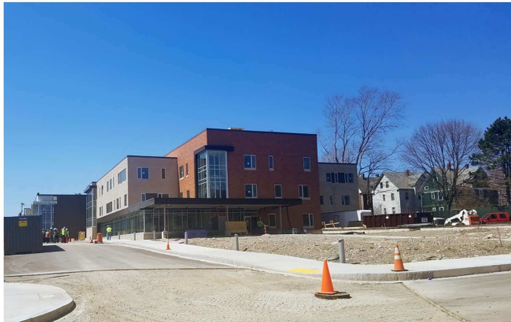
VIEW OF EXISTING SCHOOL AND FRAZER ST. RESIDENCES FROM SITE/RIVER ST.
