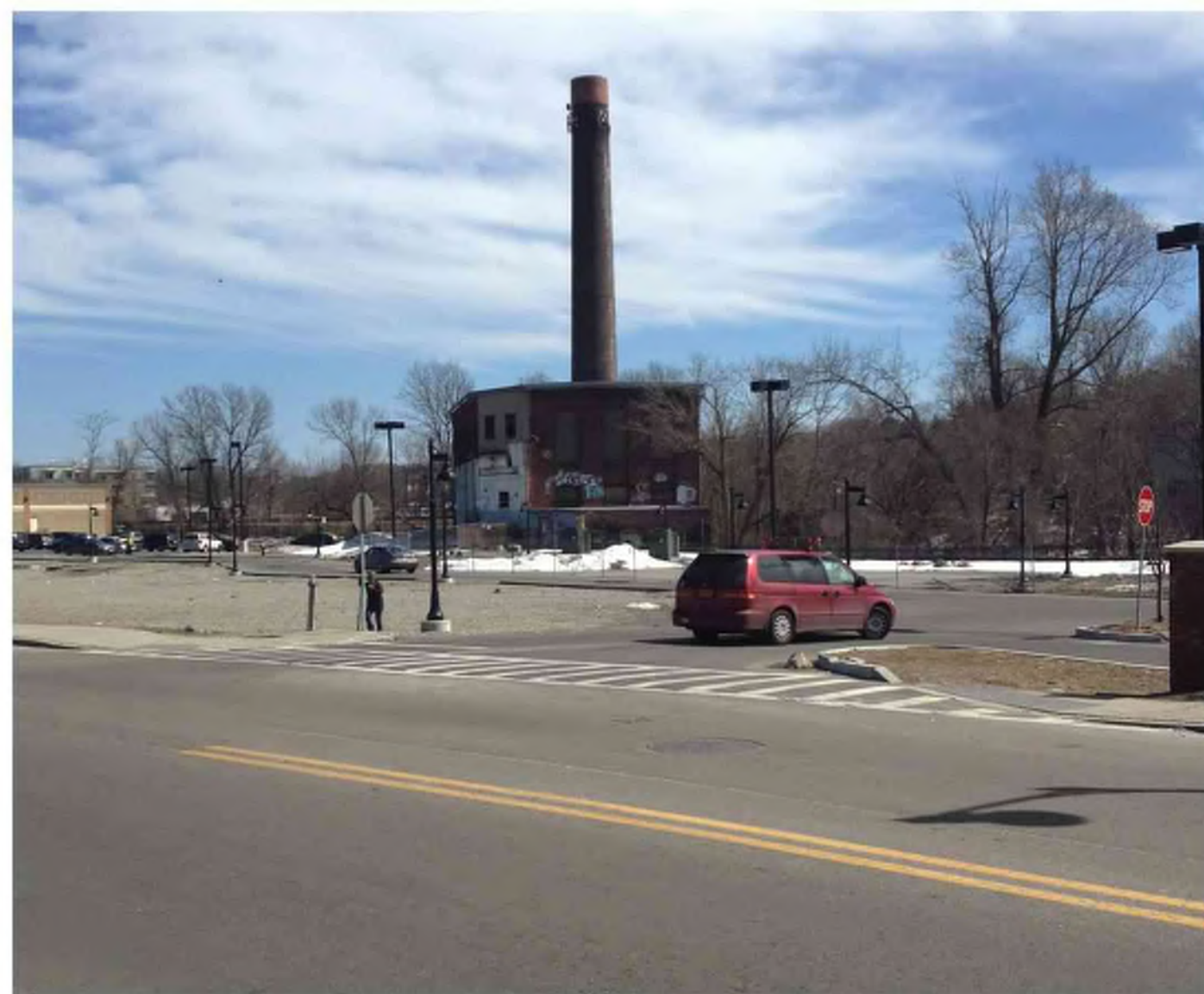
VIEW FROM RIVER ST. LOOKING SOUTH-EAST
