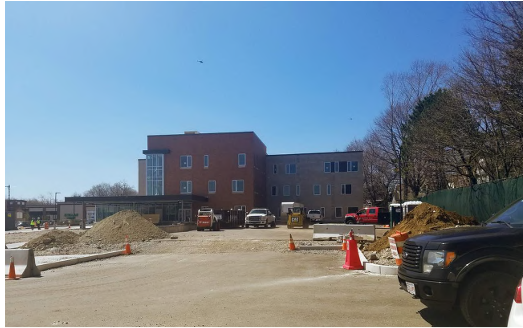
VIEW ON SITE LOOKING SOUTH-WEST
