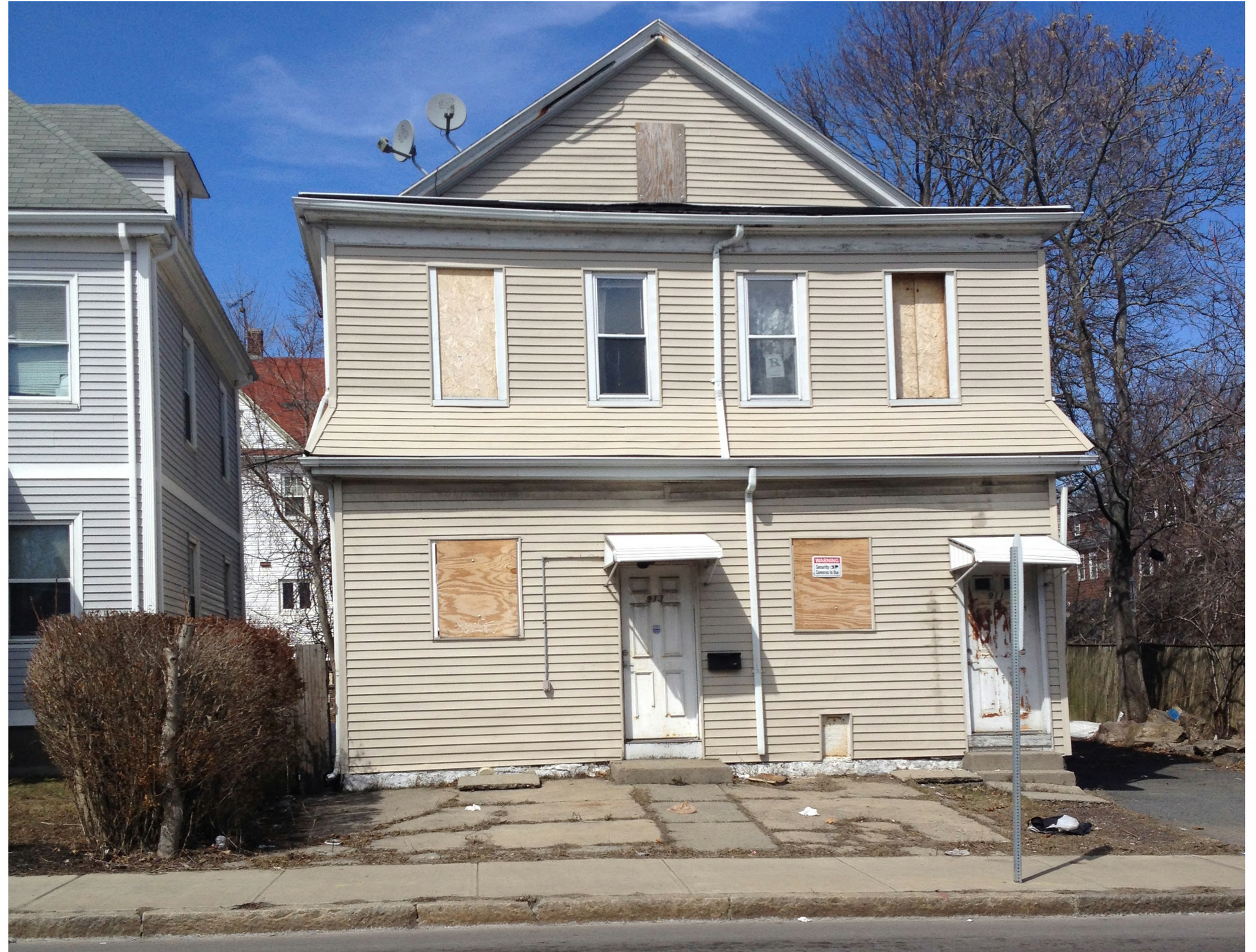
VIEW OF ABANDONED HOUSE ON RIVER ST.
