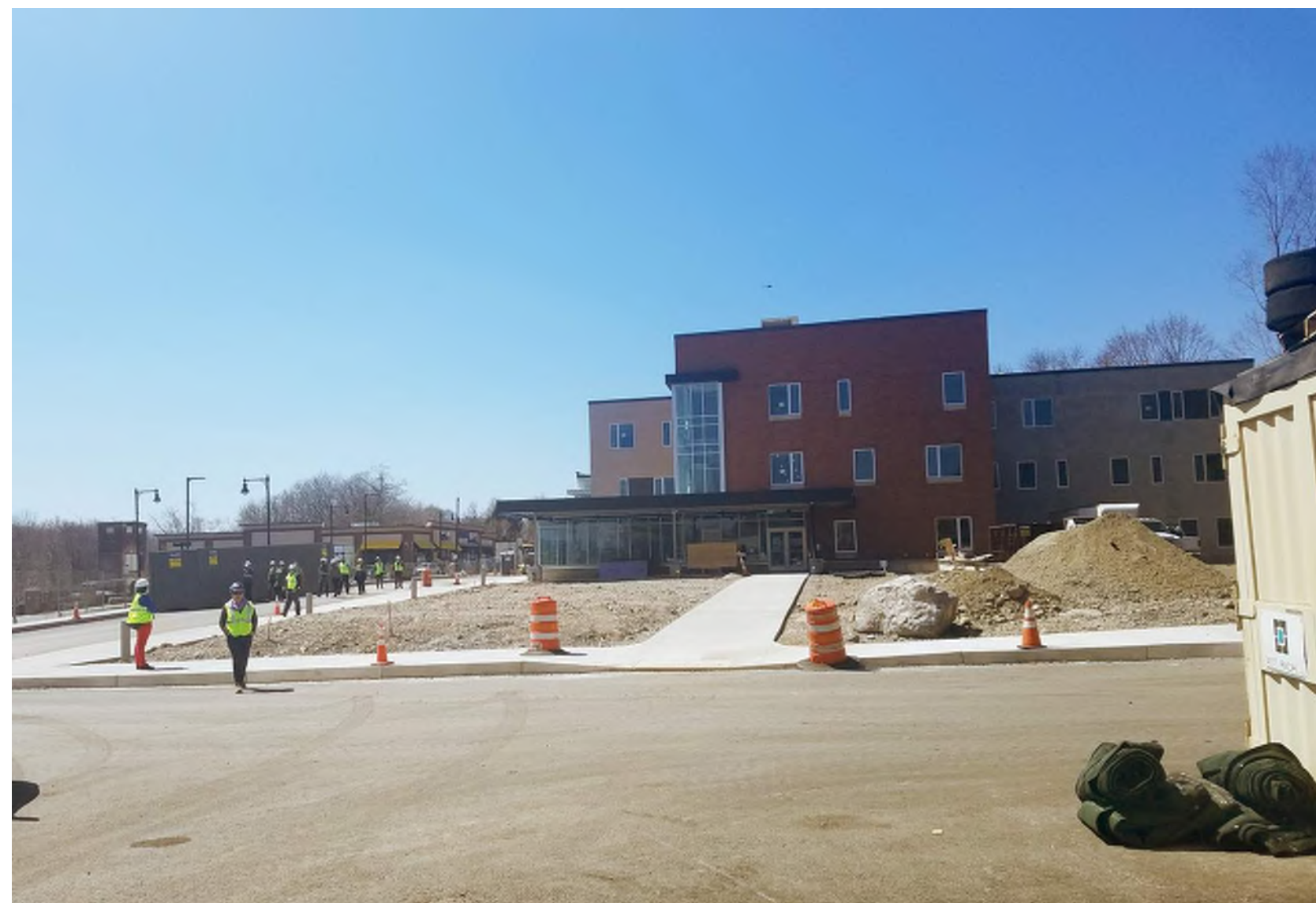
VIEW ON SITE LOOKING WEST
