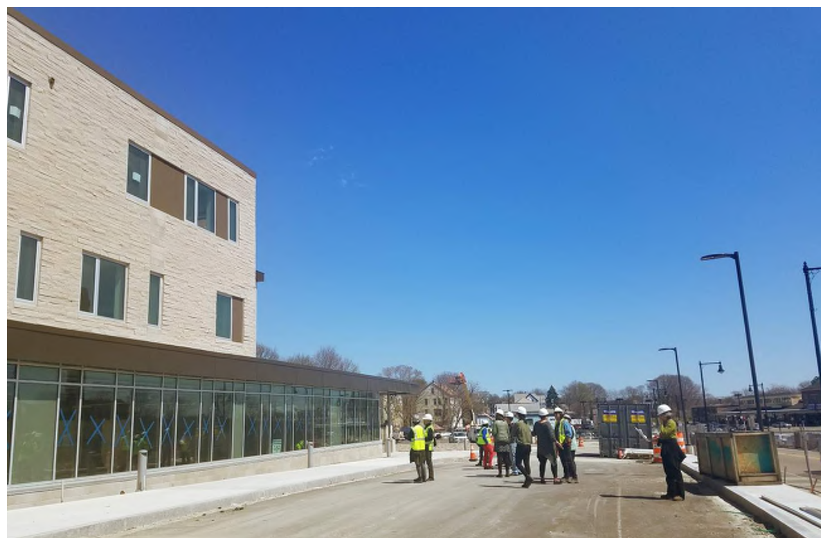
VIEW ON SITE LOOKING WEST
