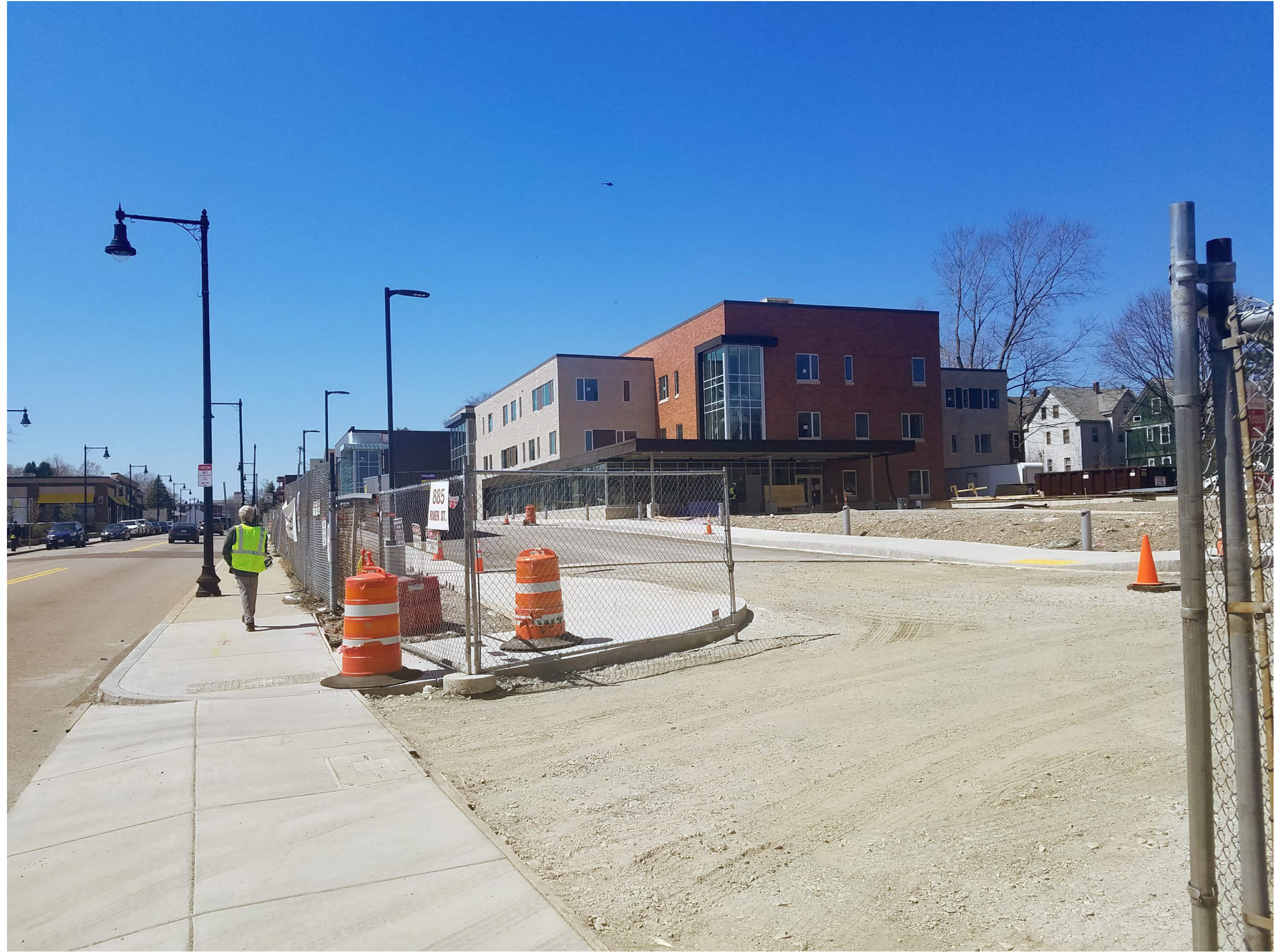
VIEW ON SITE FROM RIVER ST. LOOKING NORTH-WEST
