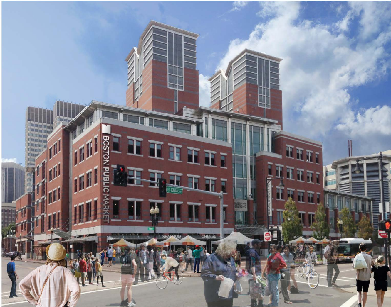
VIEW FROM HANOVER STREET AT THE GREENWAY, LOOKING NORTHWEST
