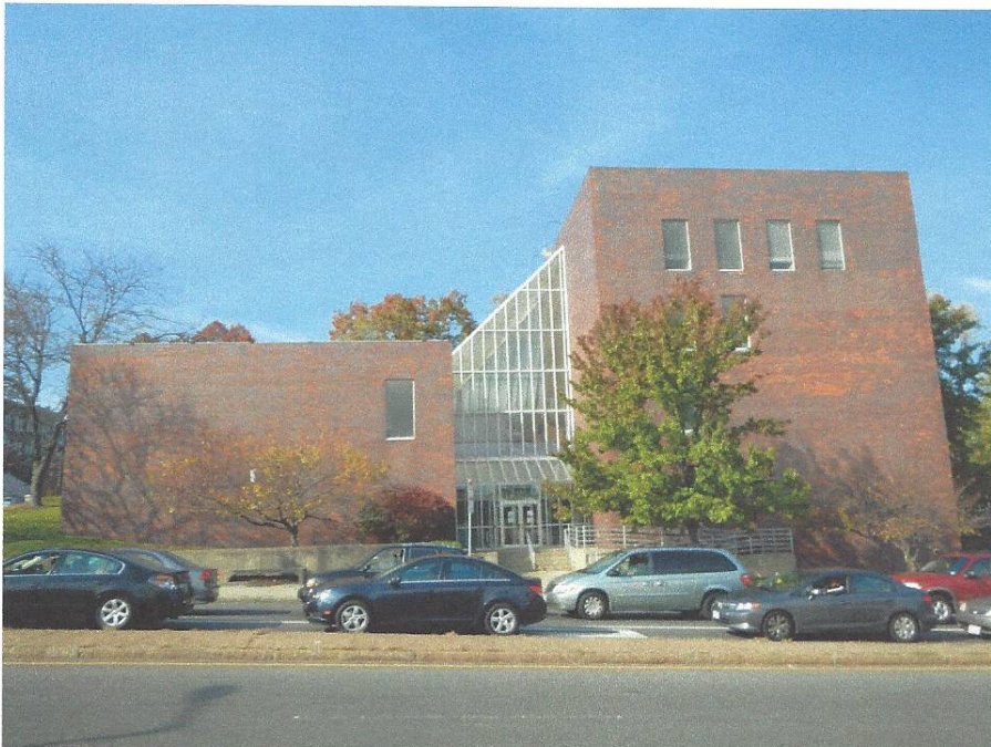
Front View of Existing Building
