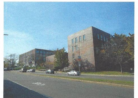
Corner View of Existing Building
