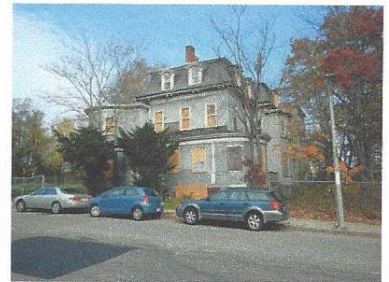
View of Existing House
