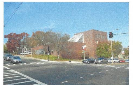
Corner View of Existing Building
