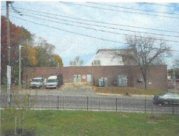
View of Existing Building
