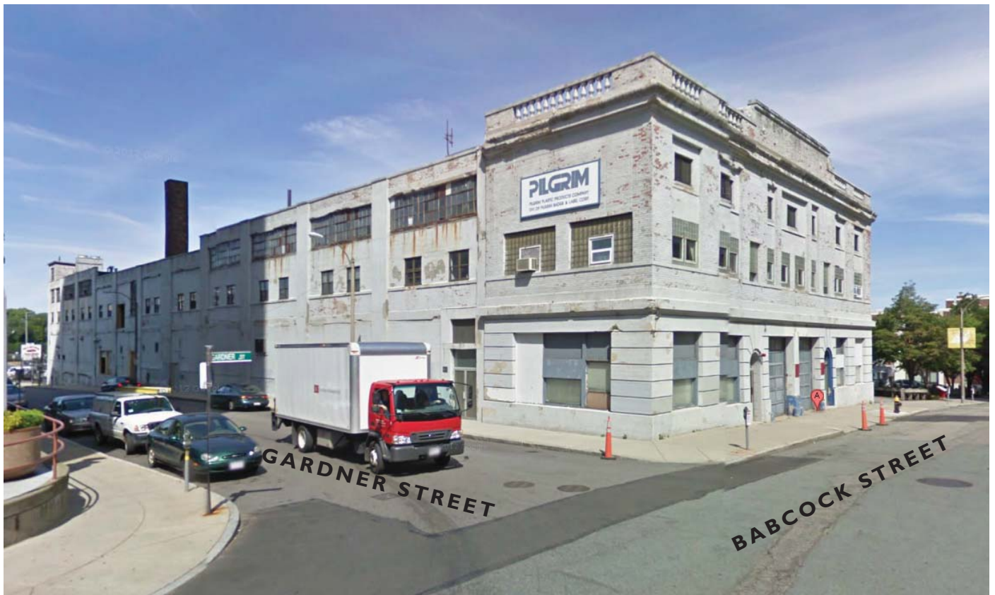
View Looking Northwest at 3-story Building
