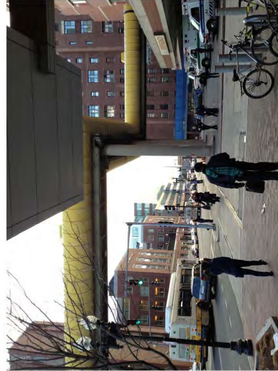
Photo 4: View from Albany St. looking southwest. Emergency Department drop-off and entrance at south face of Menino Pavilion with yellow utilities tube overhead.
