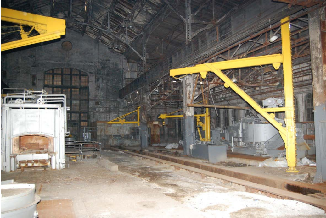
Interior View of Chain Forge Shed Atrium
