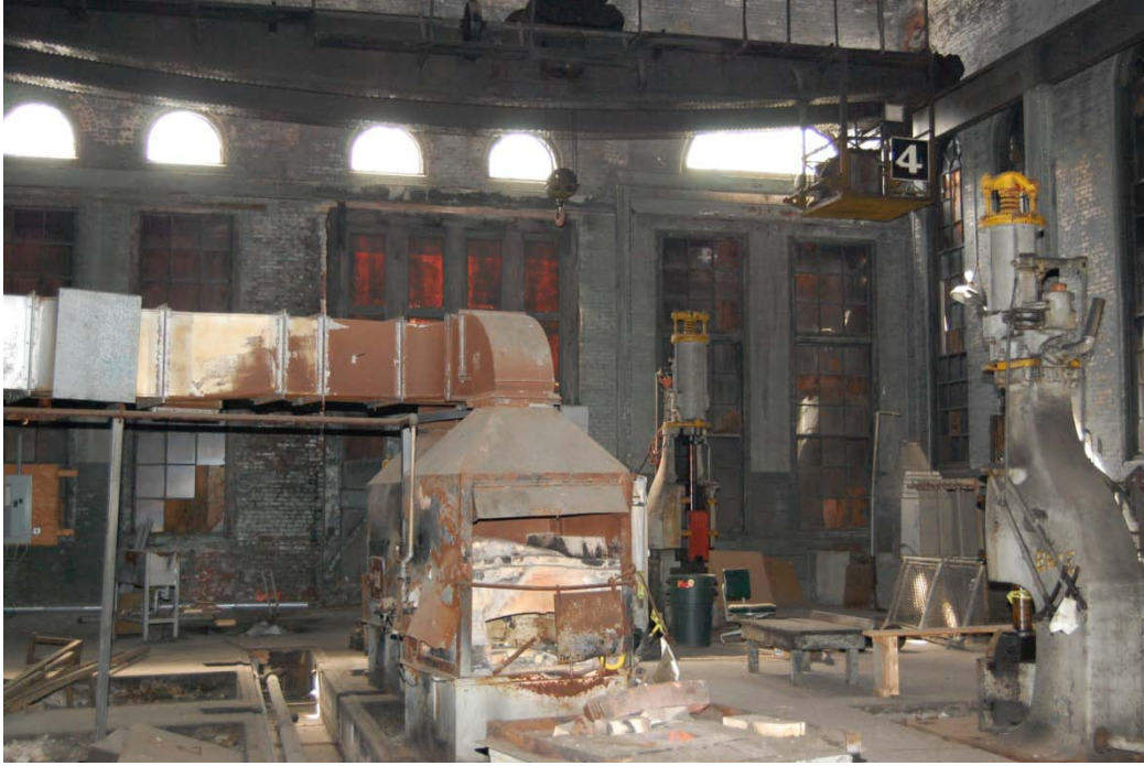
Interior View of Head House and Equipment
