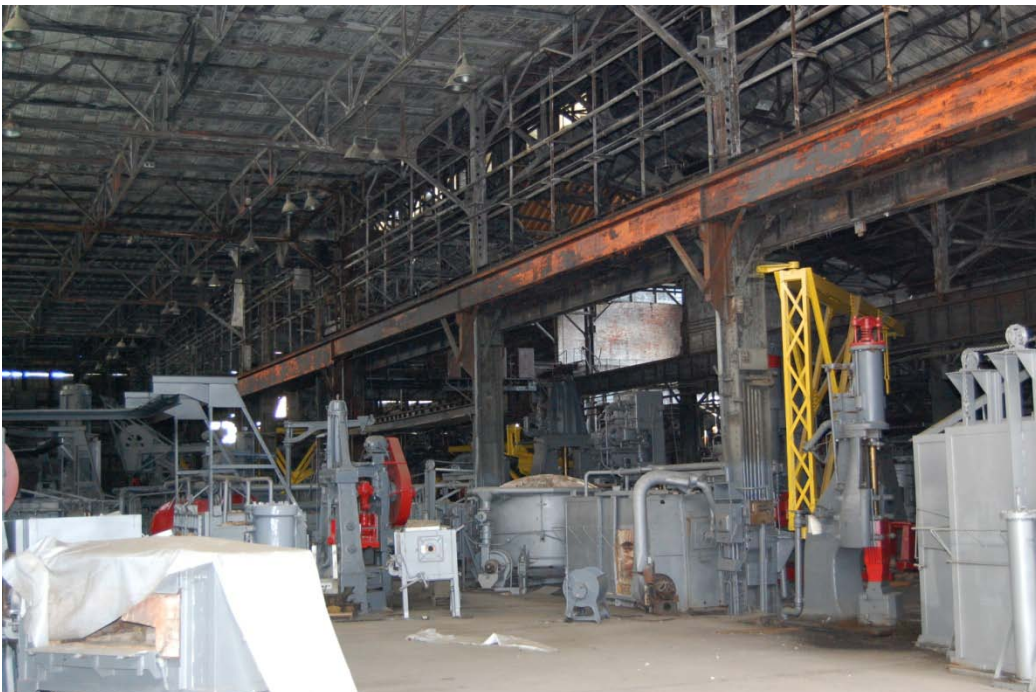
Interior View of Shed with Equipment
