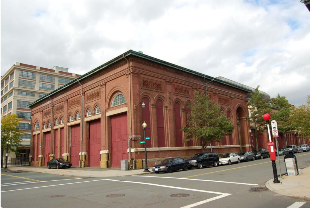
View towards Head House from corner of 1 st Ave & 9 th Street
