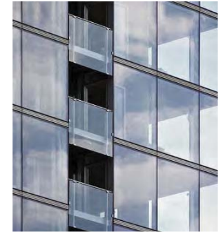
Curtain Wall Glazing
