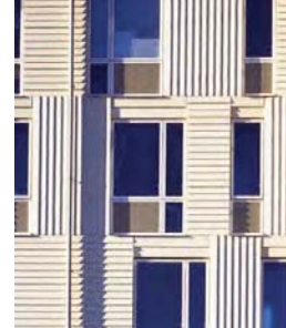
Cast Stone Rainscreen
