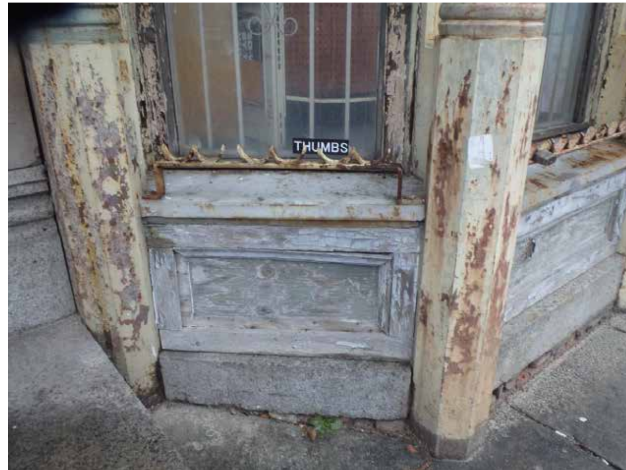
Storefront with original cast iron sill and granite base
