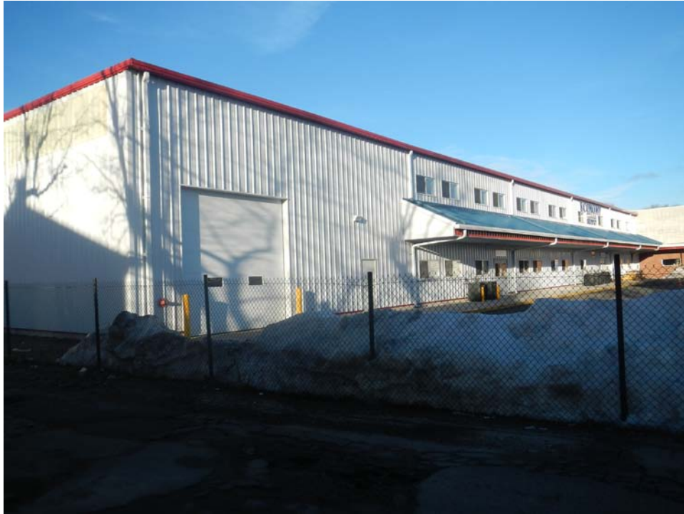
New Steel Building From Access Road Looking West
