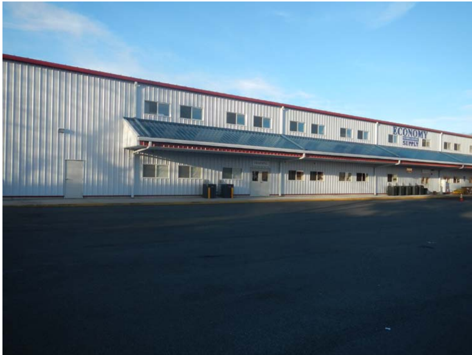
New Steel Building From Parking Lot Looking West
