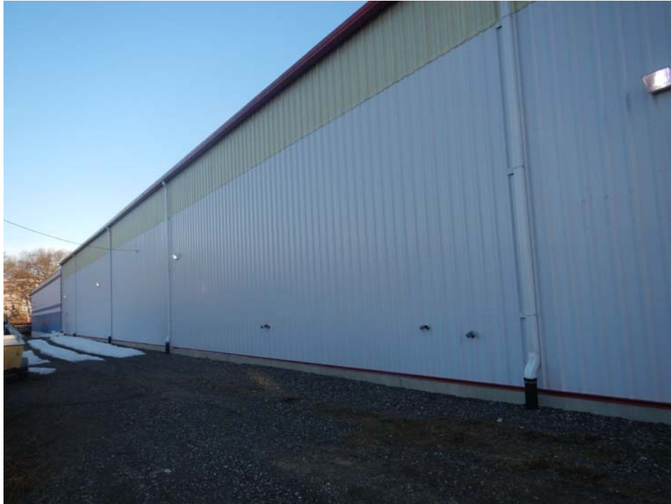
Southwest Wall of the Steel Building
