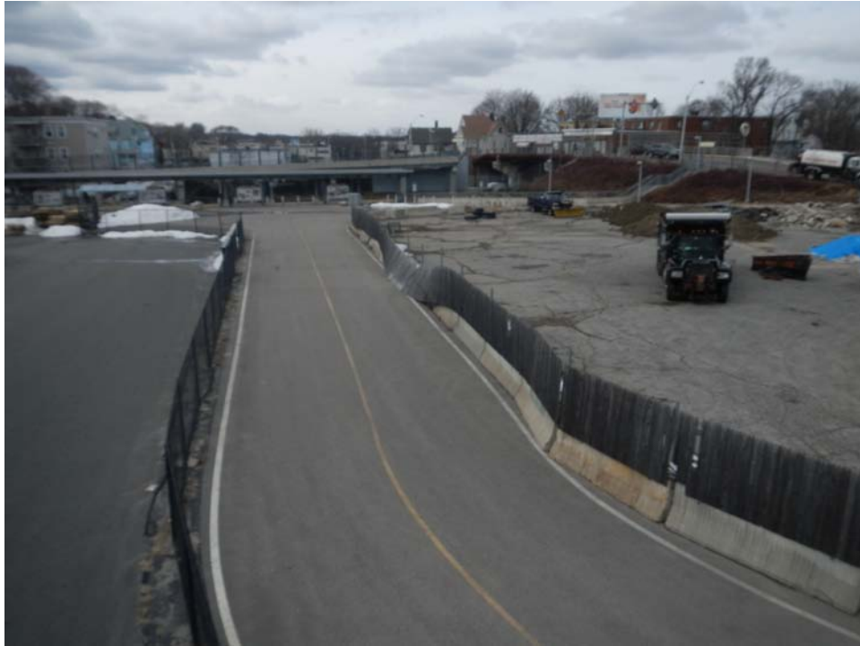
Right of Way to MBTA Station from Morton Street Entrance
