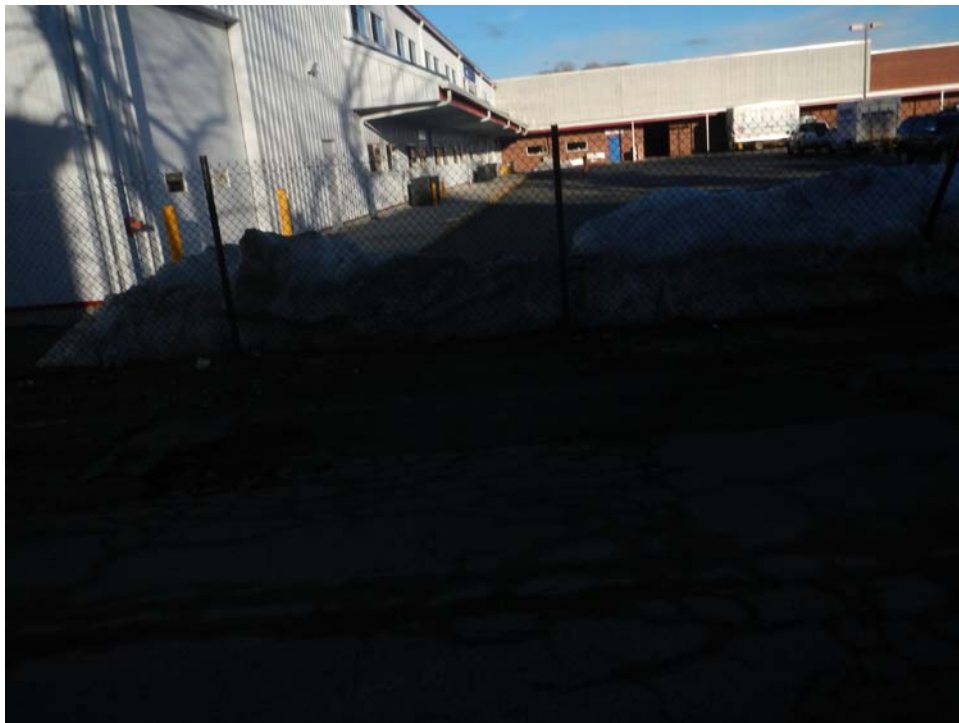
New Steel Building and Old Brick Building From Access Road Looking West
