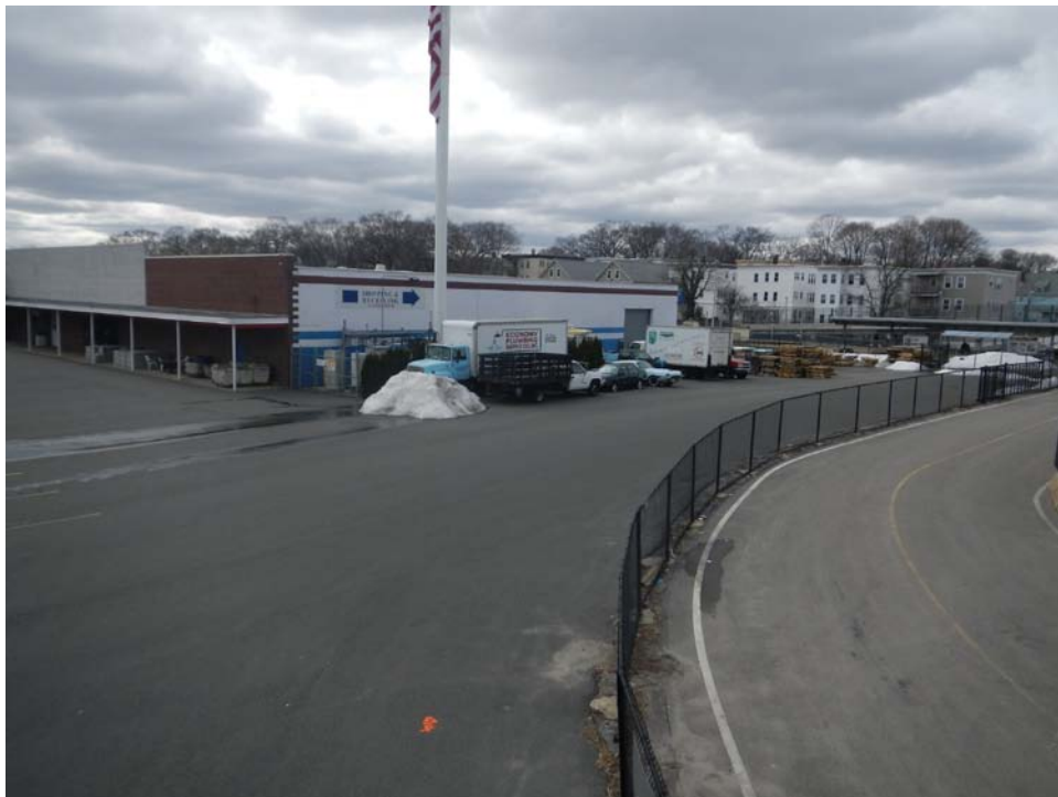
View from Morton Street Entrance Looking West
