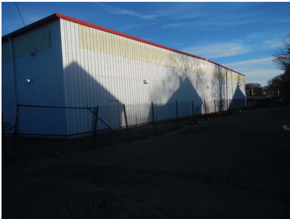
New Steel Building From Access Road Looking North
