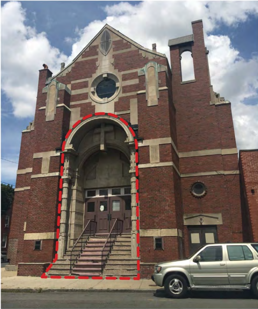
EXISTING STAIR AT CHURCH ENTRANCE
