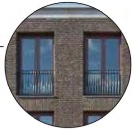
METAL RAILING BALCONY
