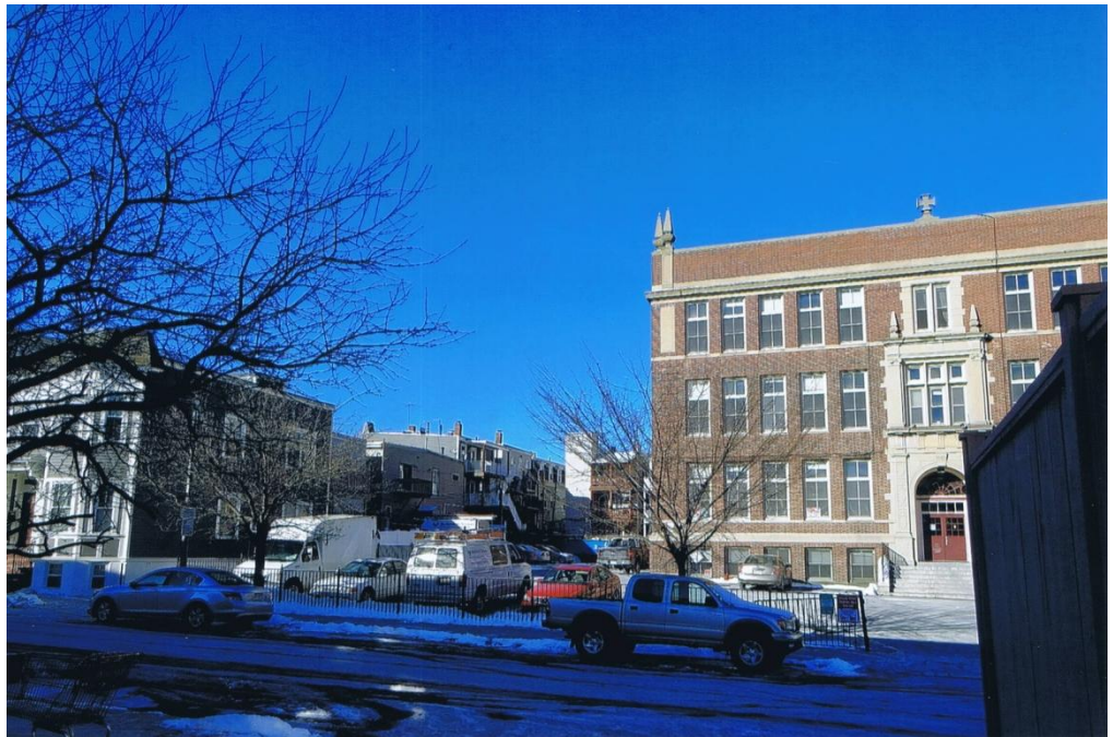
Rear Elevation – View from East 5 th Street
