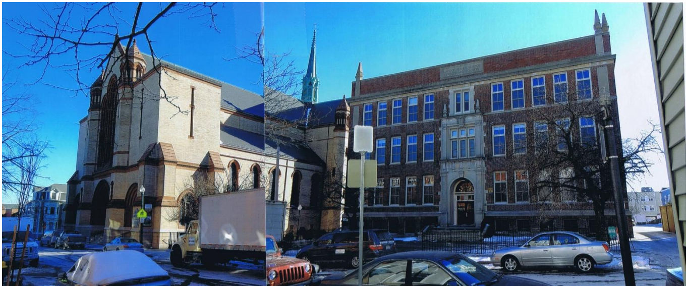
Main View of building at East 4 th Street entrance Gate of Heaven Church on the left
