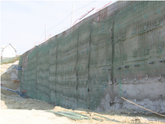
Photo #13: Reinforcement prior to final wall facing application
