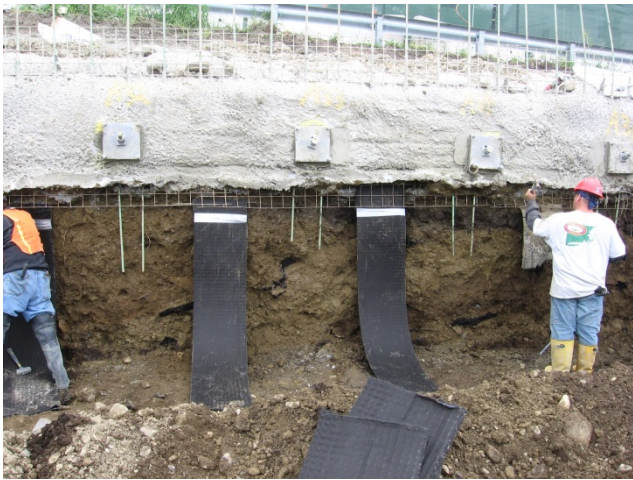
Photo #3: First layer of shotcrete and drainage strips
