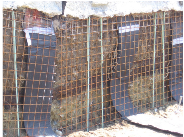
Photo #4: Reinforcement prior to shotcrete. Drainage strips in background
