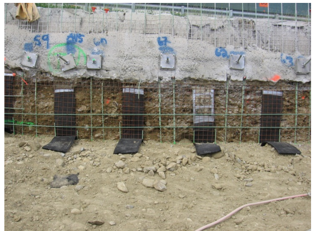
Photo #6: Soil nails, shotcrete, reinforcement and drainage strips
