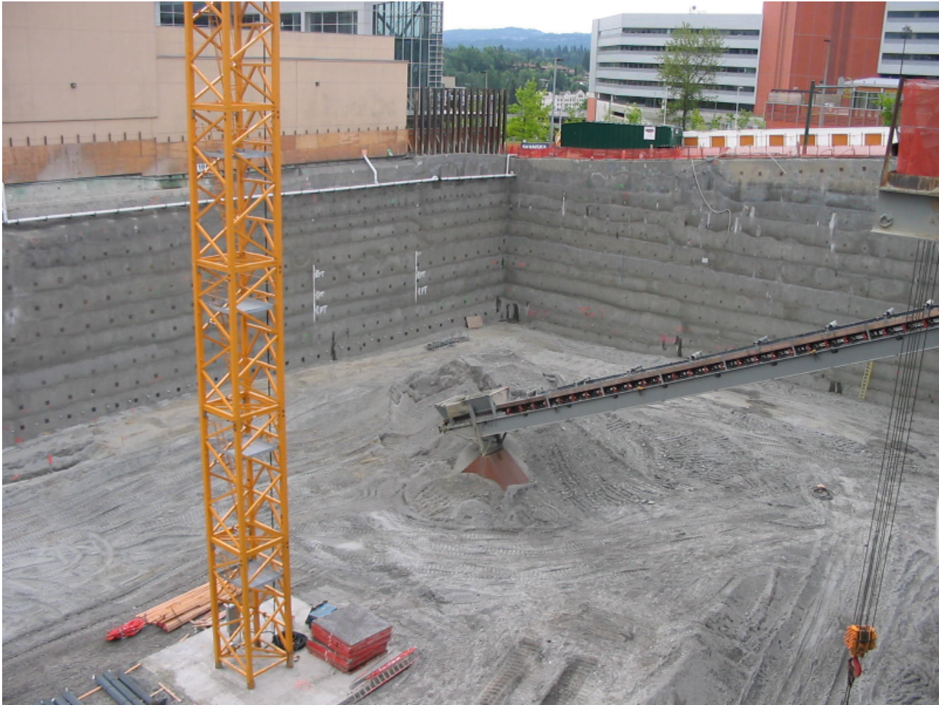
Figure 1. View of Bravern Excavation toward Meydenbauer Convention Center.
