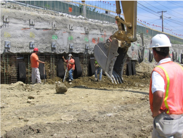
Photo #7: Second layer of shotcrete
