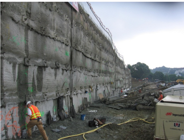
Photo #11: Drilling final row of soil nails
