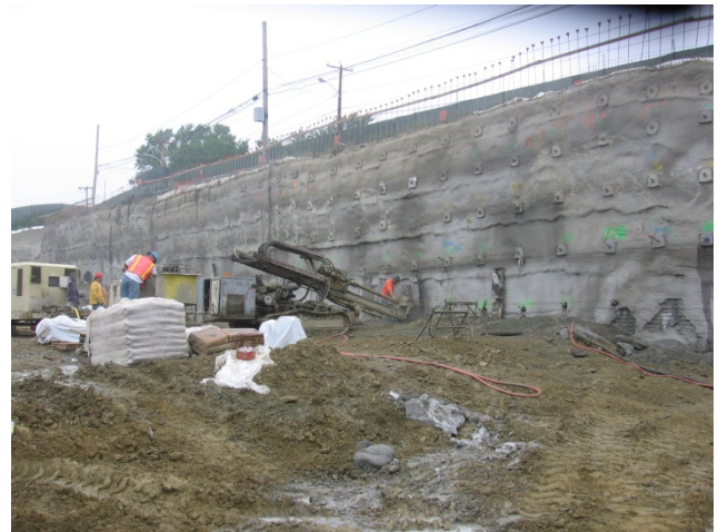
Photo #10: Drilling of soil nails
