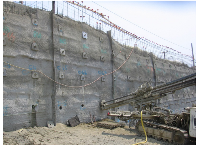
Photo #8: Drilling of soil nails
