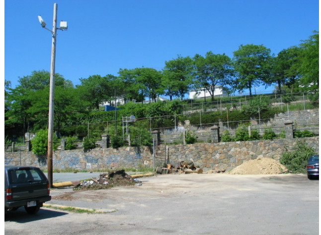
Photo #2: Site before construction
