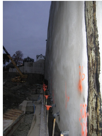
Photo #16: Side view of wall (nearly vertical)
