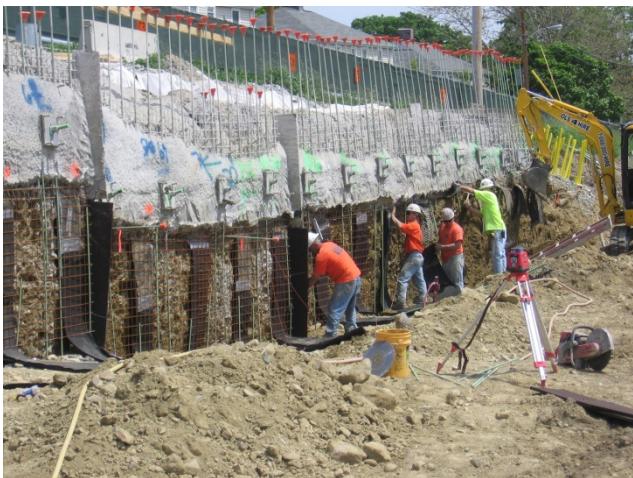
Photo #5: Prepping wall for shotcrete
