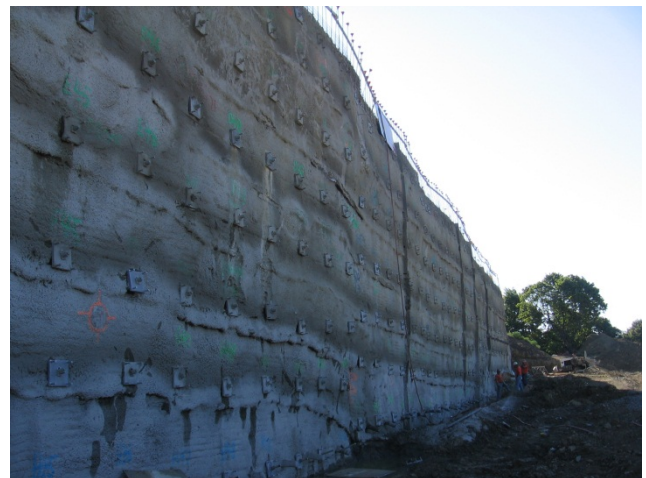
Photo #12: Completed wall prior to final facing
