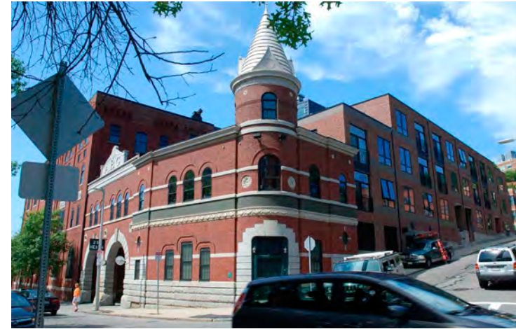
30. View of American Brewing Company building (BOS.7827) from the intersection of Heath Street and Estey Street, facing NW.
