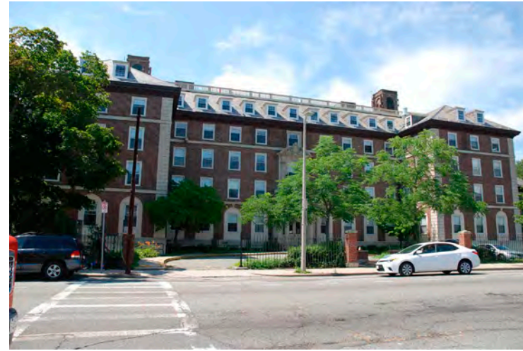
2. View of Goddard House, east façade, facing NW.
