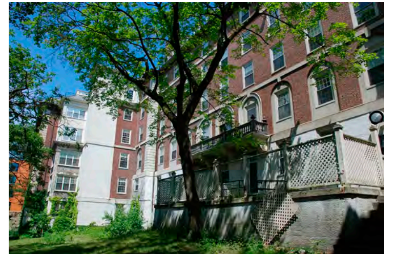
8. View of west (rear) elevation of Goddard House, facing NE.
