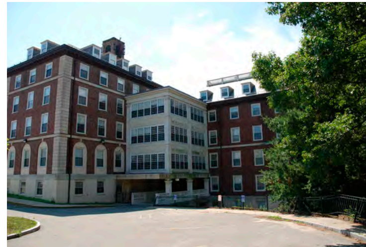
7. View of connection between Goddard House and 1931 addition, facing SW.
