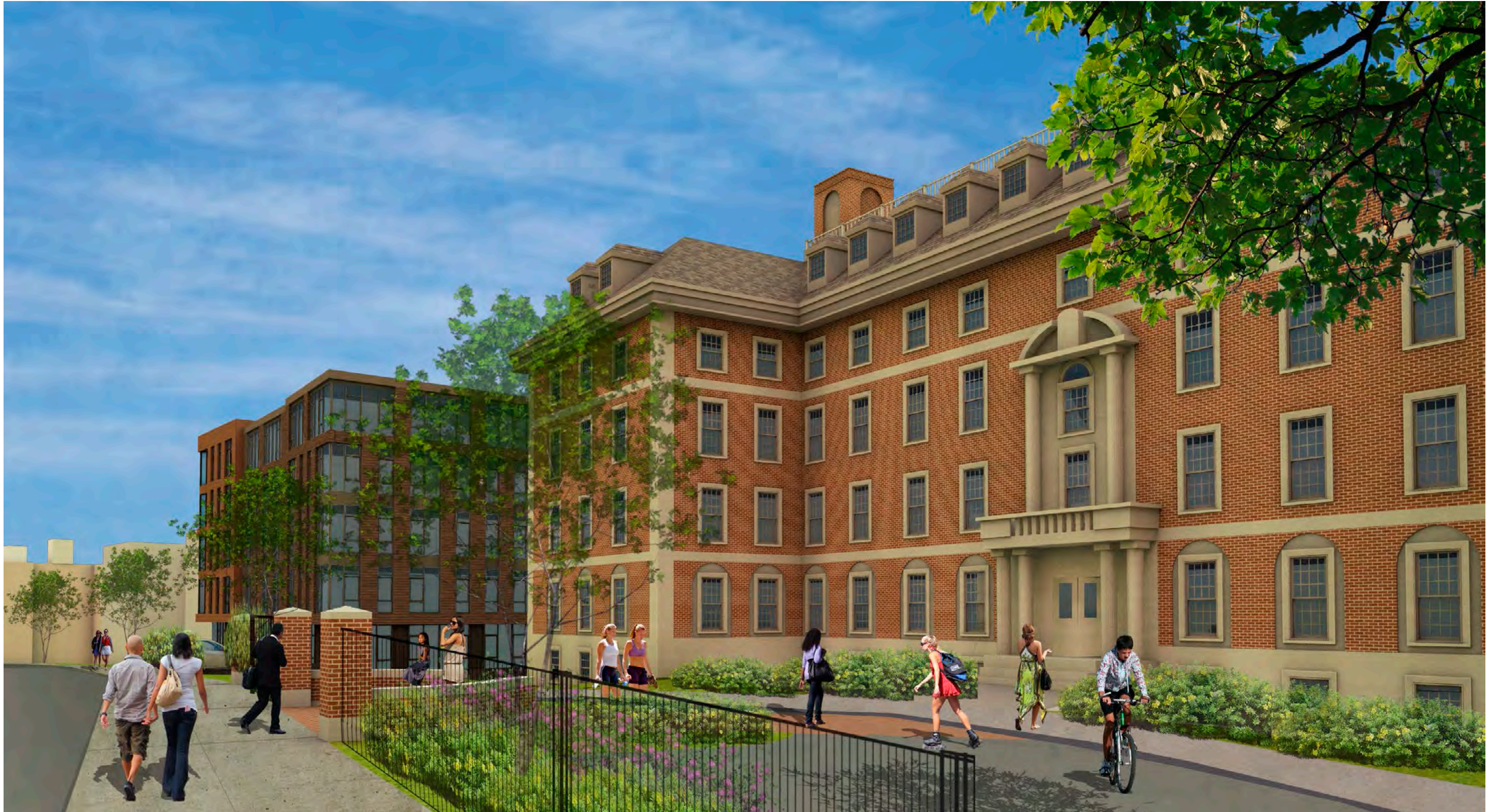
View of Goddard House looking south on South Huntington Avnuuee
