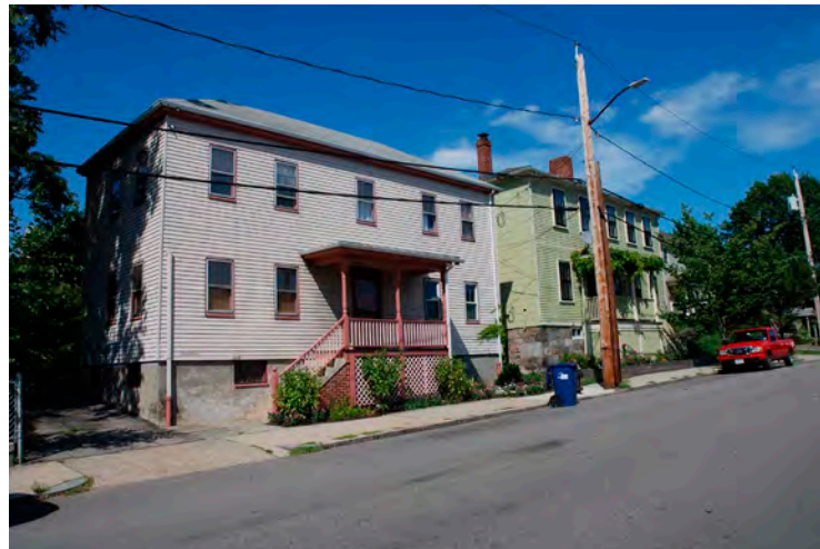
32. View of 33 and 47 Bynner Street (BOS.7734 and BOS.7735), facing NE.
