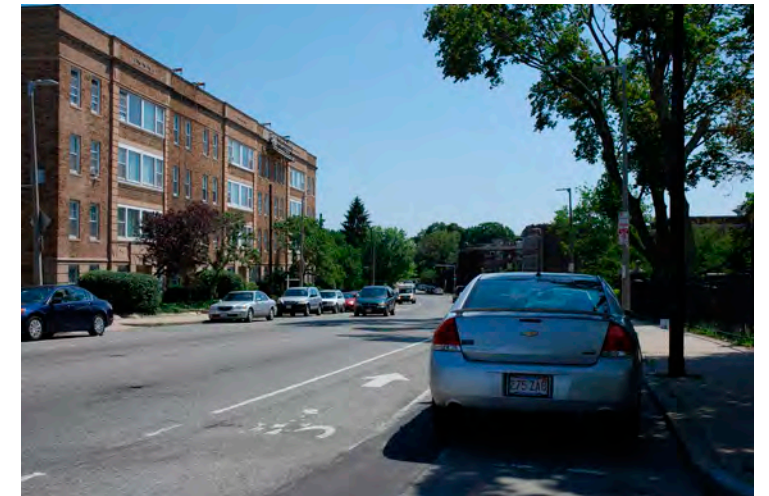
16. View of South Huntington Avenue streetscape south of Goddard House, facing S.
