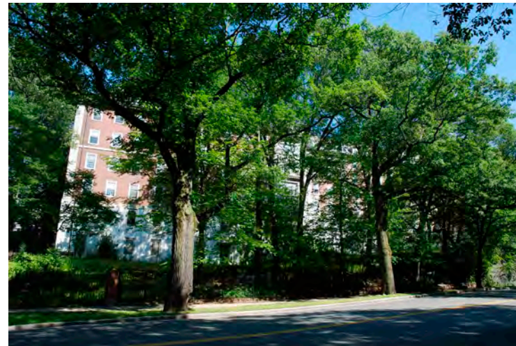
22. View of Goddard House west elevation from the Jamaicaaway, facing SE.
