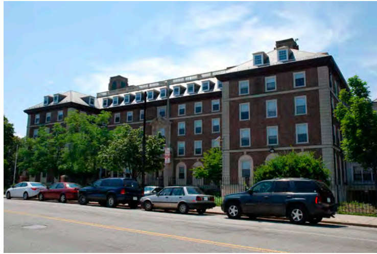
1. View of Goddard House, east façade along South Huntington Avenue, facing SW.
