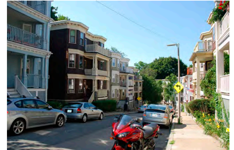
31. View of Parkton Road streetscape (BOS.JI), facing N.
