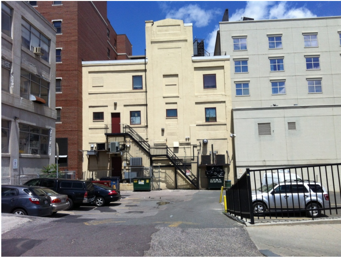
Rear of 530 Commonwealth Avenue from Newbury Street
