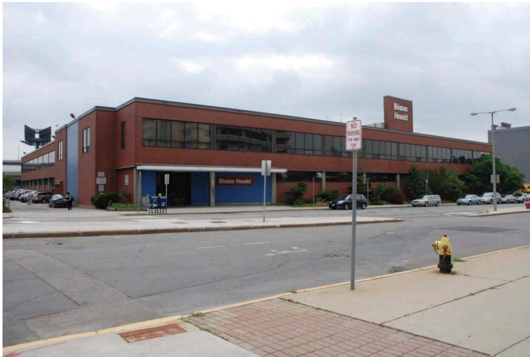
1. Herald Square Project, 300 Harrison Avenue, Boston, MA. View of front (west) and north side of Herald building. Photographer facing SE, June 2011.
