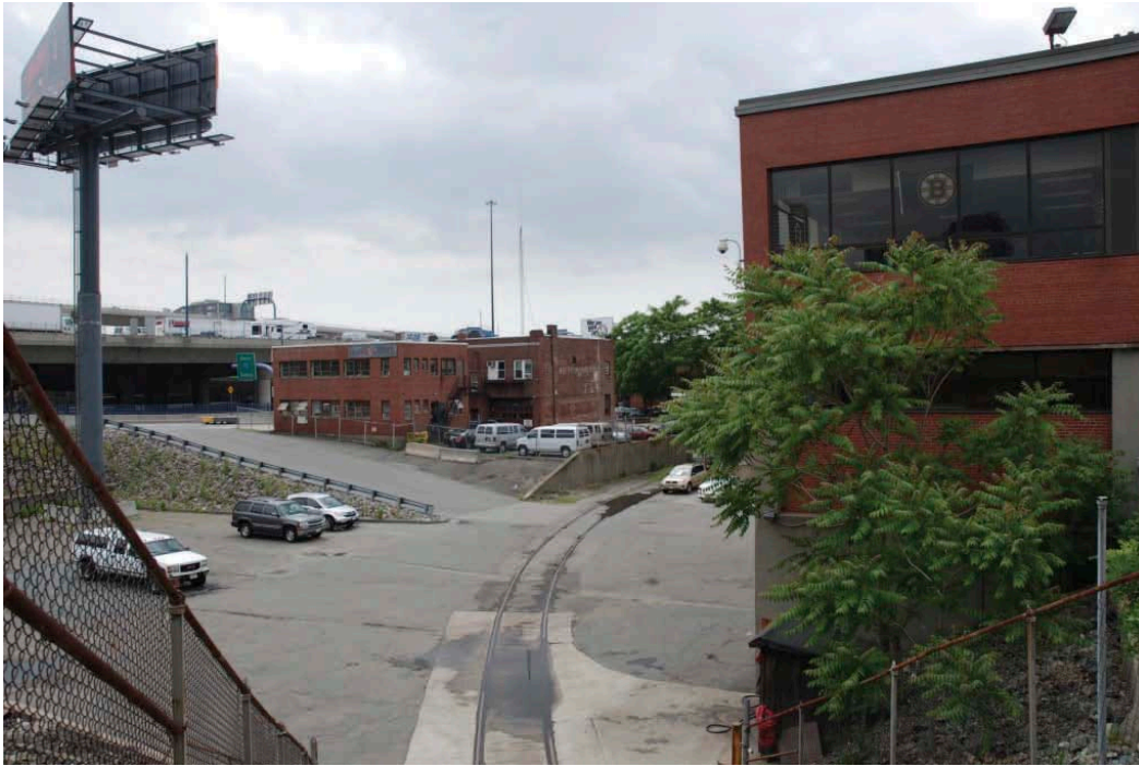
11. Herald Square Project, 300 Harrison Avenue, Boston, MA. View of 217 and 233 Albany Street in rear and Herald building on right, from Herald Street. Photographer facing SE, June 2011.
