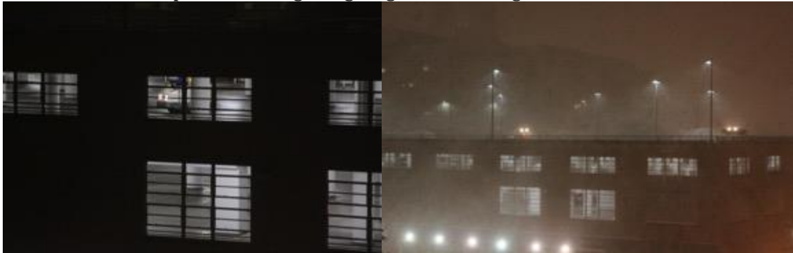
Exhibit 2.1 and Exhibit 2.2/2.3: Parking Garage Being Cleaned at 11:17 PM and Bobcats and Caterpillar clearing the garage and loading dock at 2 am
