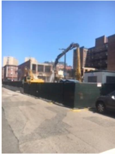
Exhibit 5.1: Current construction adjacent to 16 Miner St.
