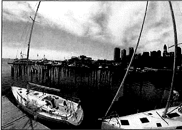
Photo 2 - 2015/08/05 1100 hrs. Approximately 126 Piles In View Low Tide 0943 hrs. (-1.0 Feet)
