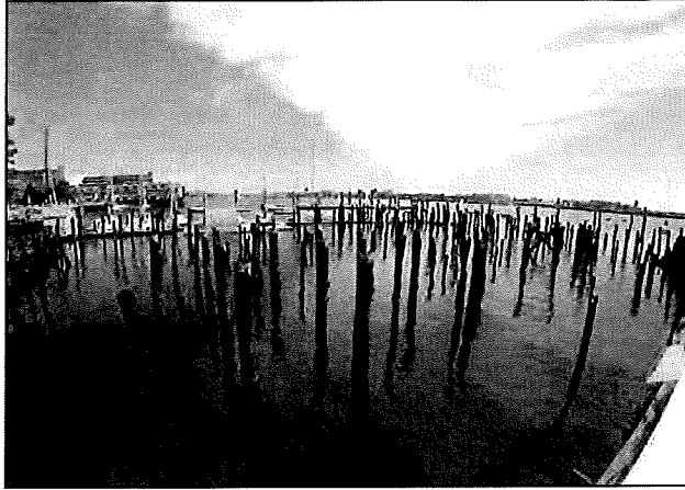
Photo 2 - 2015/08/05 1100 hrs. Approximately 160 Piles In View* Low Tide 0943 hrs. (-1.0 Feet)
